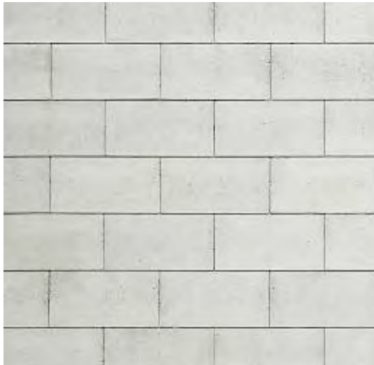
WHITE PAINTED CONCRETE MASONRY UNITS, ON ALLEY ELEVATION
