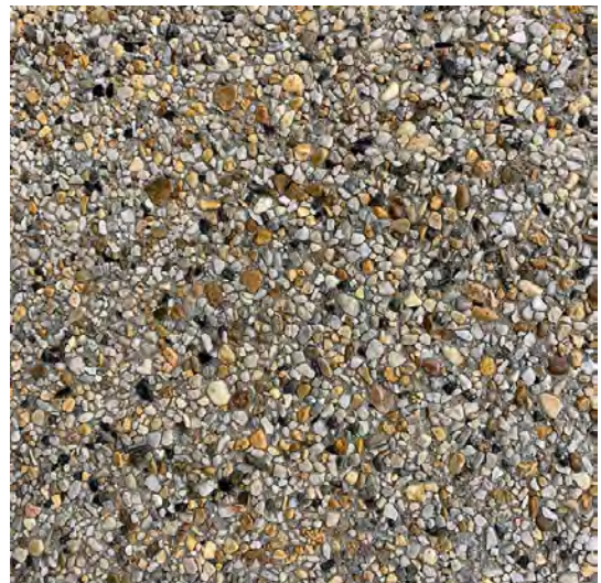
EXPOSED AGGREGATE CONCRETE RAMPS, LANDING & APPROACHES AT OLD WOODWARD STOREFRONTS
