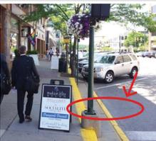
As displayed in the image to the left, a stepped curb is located in numerous areas in the downtown. These can present hazardous situations for some pedestrians, especially when they are located at crosswalks where there are no ramps. The near-term recommendation is to remove the stepped curb by installing curb ramps at road crossings. In the long-term the stepped curb should be eliminated throughout the downtown by re-grading the road.
