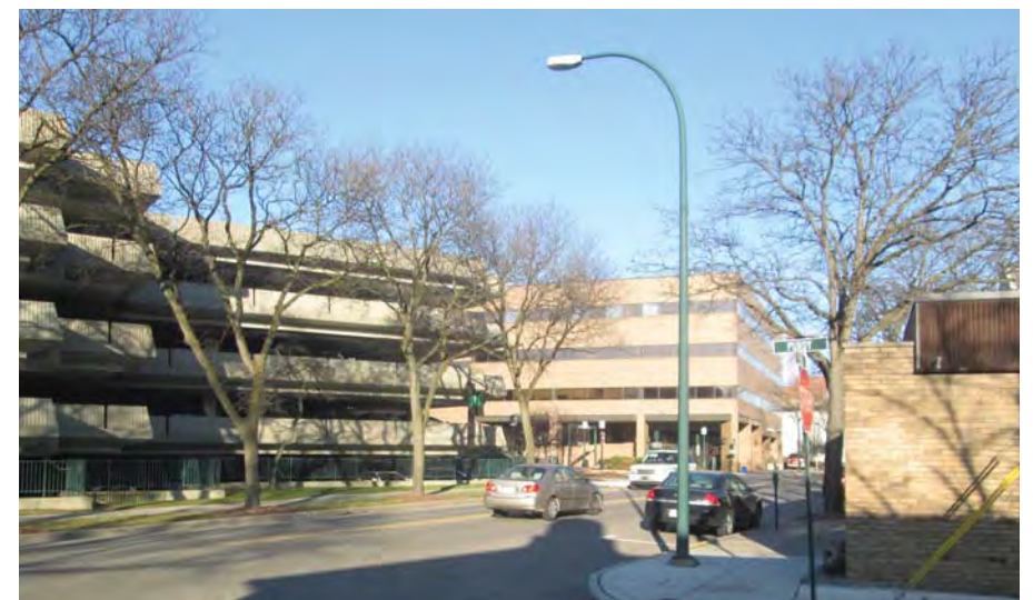
PIERCE PARKING DECK EXPANSION BIRMINGHAM, MICHIGAN JANUARY 12, 2015
