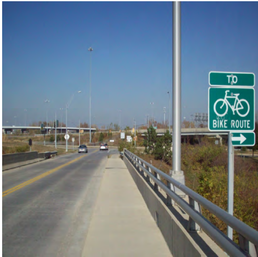
Figure 2. Five-foot-wide sidewalk designated as section of two-way multi-use path on Souder Ave. bridge (Columbus, OH). (Photo: Ariel Godwin.)
