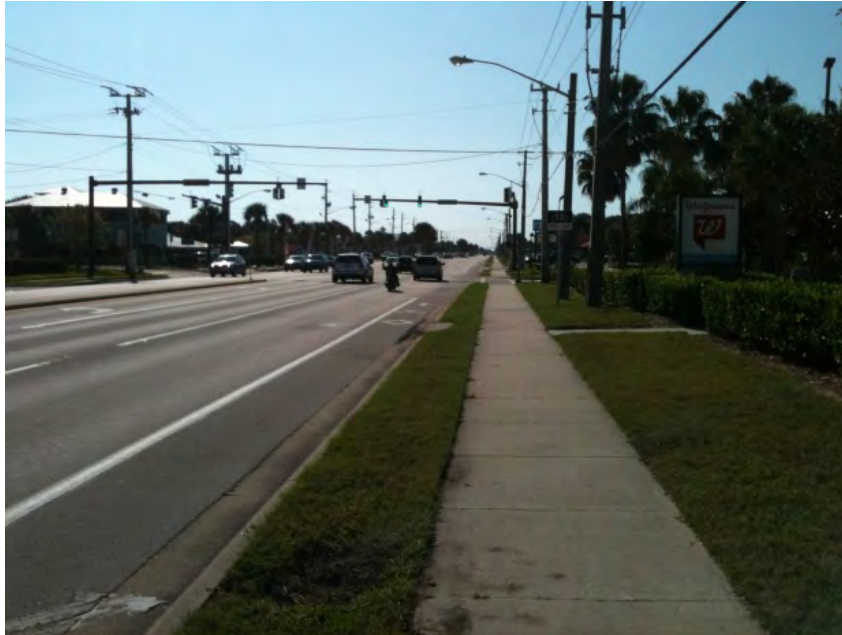
Figure 1. Arterial road in Florida with bike lane adjacent to high-speed traffic and gutter pan partly occupying bike lane. Some cyclists may perceive the sidewalk as safer. (Photo: Ariel Godwin.)
