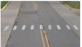
Paint pavement marking is the most widely used material in pavement markings in Canada and the United States.
