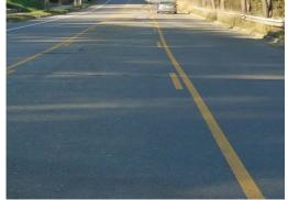
may not provide a sufficient chemical bond between asphalt and the thermoplastic marking material. Thermoplastics provide excellent performance when applied properly. The service life of thermoplastic marking paints normally ranges between forty eight months and eighty four months depending on different factors including application procedures, pavement type, traffic volume, snowplow activity and atmospheric conditions when placed.
