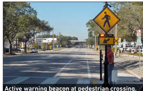
Active warning beacon at pedestrian crossing.
