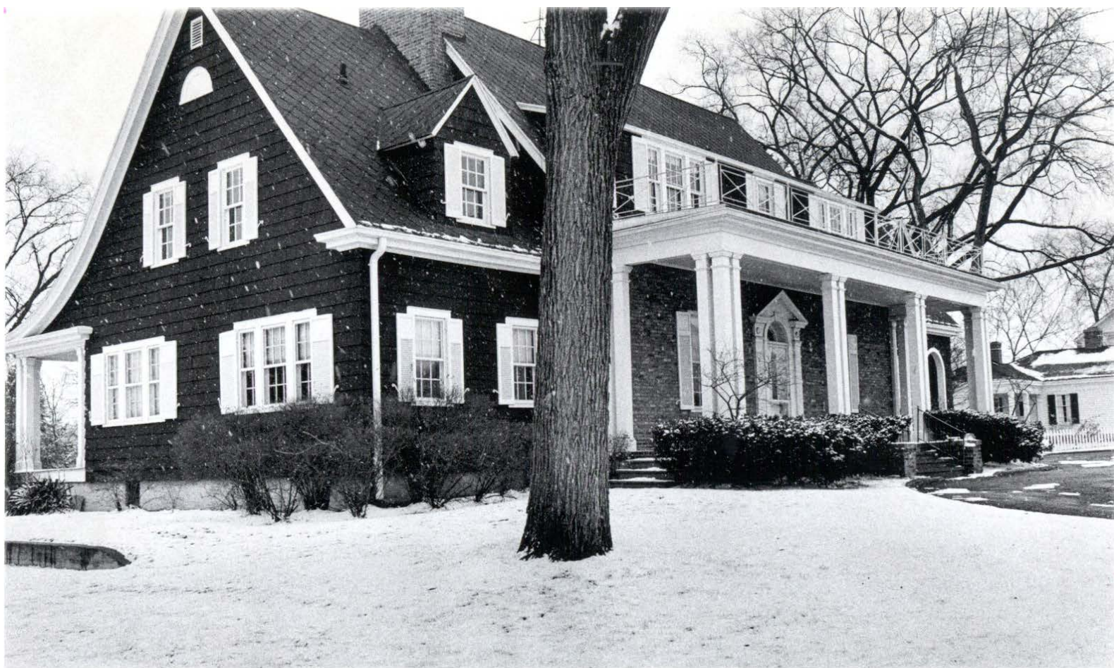
Allen House 2001, showing old asphalt roof and cedar shingles, with newer railing above porch.
