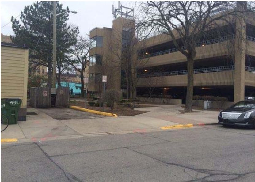
The scruffy concrete spot beside a car park has been used for pop-up concerts, and now city officials have plans for high-tech features. (Photo: City of Royal Oak)
