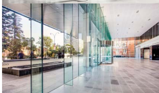
STRUCTURAL GLAZING WITH GLASS FINIS
