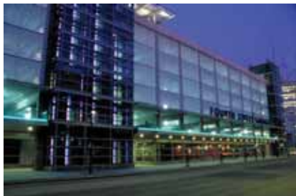
Precast panel and glass louver screening, plus photovoltaic panels on top deck (upper), and metal screen with tower element marking the entry corner and vertical circulation (lower).
