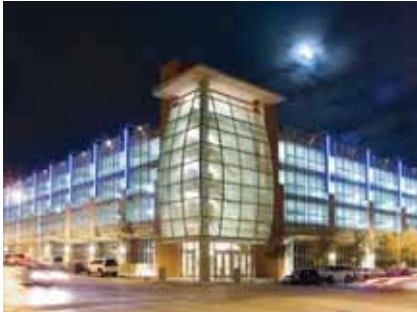
Precast panel and glass louver screening, plus photovoltaic panels on top deck (upper), and metal screen with tower element marking the entry corner and vertical circulation (lower).
