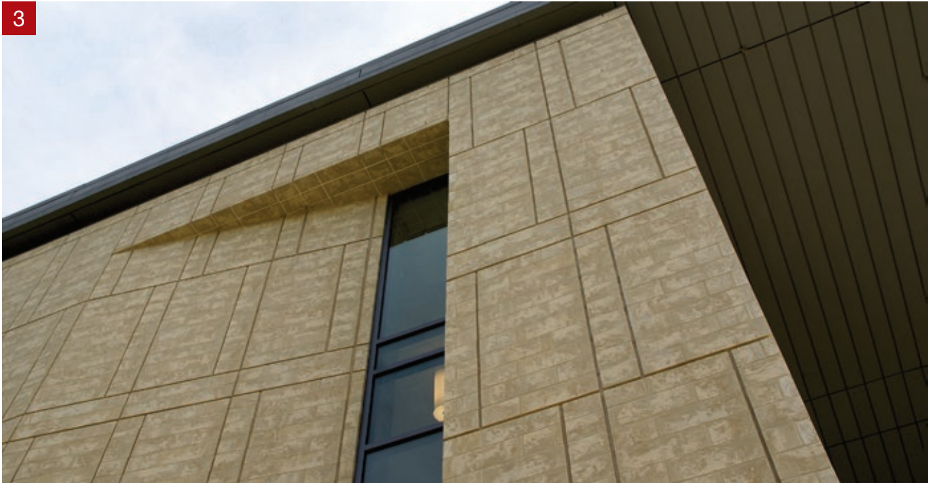
1. Custom Arch and Post units, Bullnose | 2. Bullnose and custom detail | 3. Notches to emulate large panels
