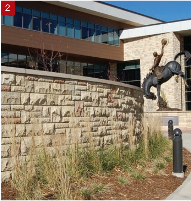
1. Stone installed in a vertical quarter bond pattern | 2. Blend of standard colors (Suede, Café, Garnet) installed in an ashlar pattern.
