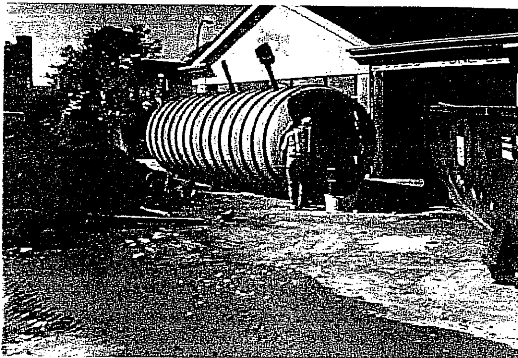
The USTs being cleaned.
