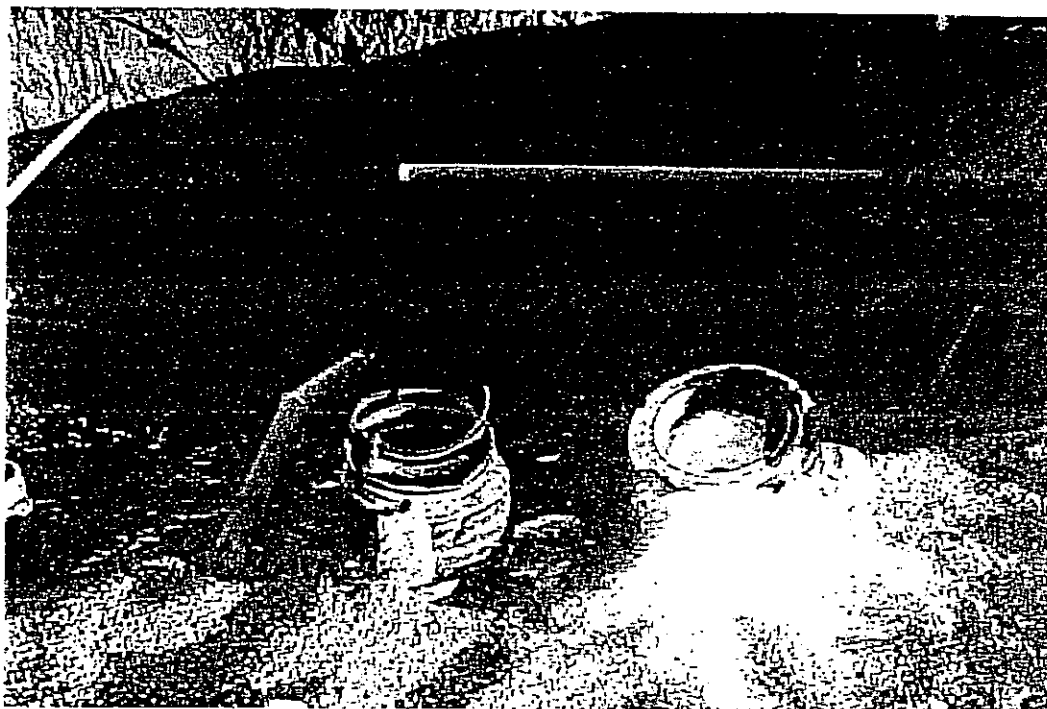
Dry ice being used to inert USTs.
