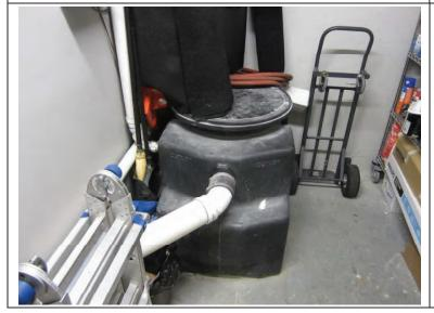
**Photo 9.** Oil-water separator in connection with elevator in basement level of Property building
