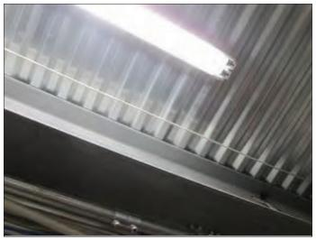
19. Metal deck and steel beam of second floor
