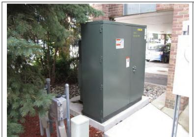
**Photo 10.** Pad-mounted transformer on western Property boundary
