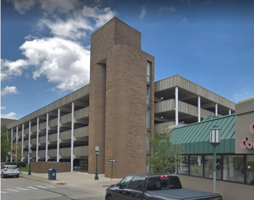
Park Street Parking Structure
