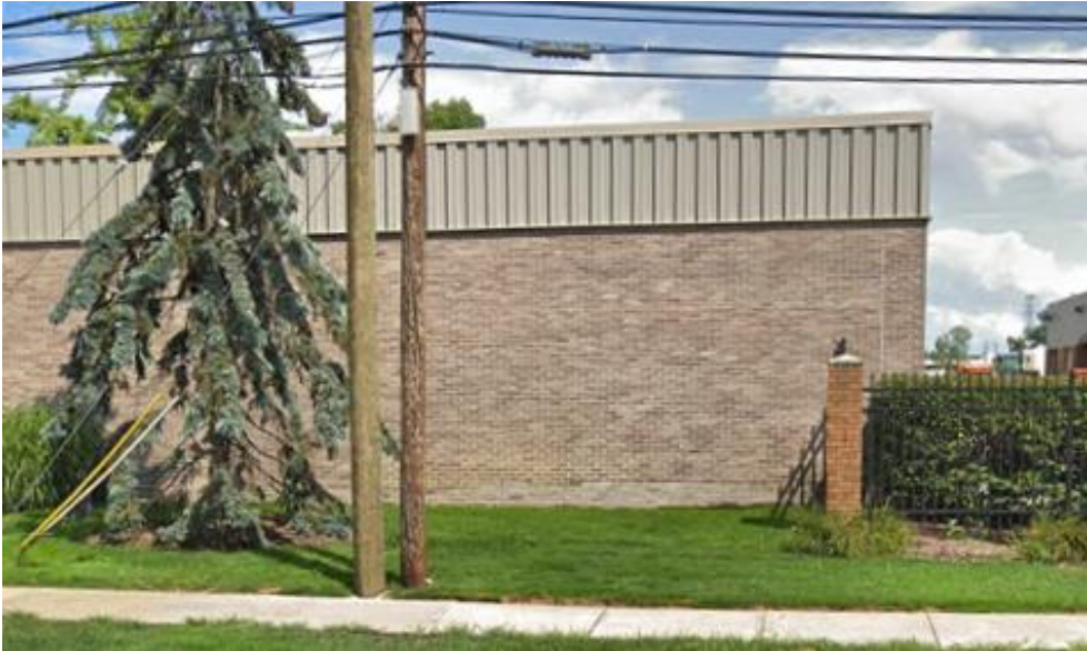
3.) DPS Building facing Eton Street
