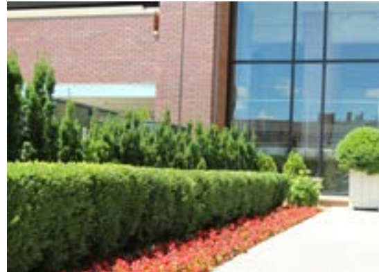
Utility boxes screened by shrubs
