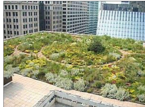
Green Roof in Chicago
