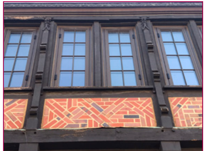
Maintenance and repair of original wood exterior details is key. The wood in the image above requires some repair from water damage and repainting. City of Birmingham, photo by KDG, 2022.
