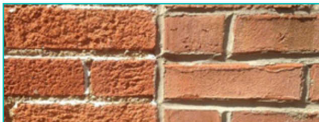
Sandblasting and other abrasive cleaning methods will severely damage historic masonry as seen here at left. The hard exterior shell of the brick, known as the fire skin, has been destroyed. This brick will begin taking on water and will deteriorate quickly. City of Birmingham, photo by KDG, 2022.
