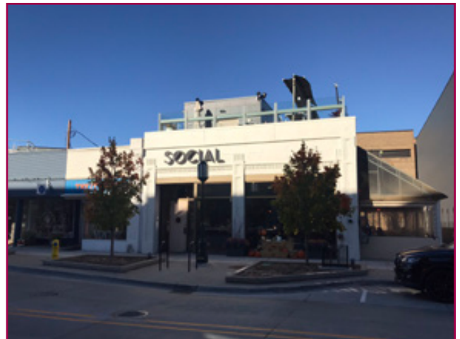
It is not recommended to build additions that are visible on the primary facade. Here both the rooftop railing and canopy are highly visible as is the addition on the side of the building. City of Birmingham, photo by KDG, 2022.
