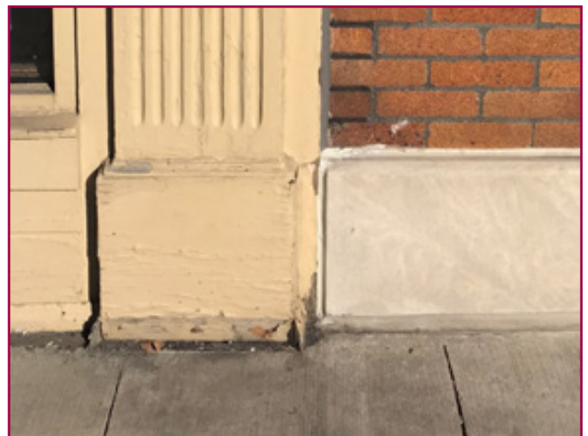
Peeling exterior paint and missing wood trim are indicative of needed maintenance, City of Birmingham, photo by KDG, 2022.
