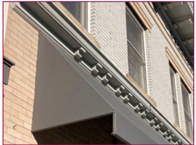
Close inspection, repeatedly completed, is key for a preventative maintenance plan. This storefront is missing modillions, likely a result of deferred maintenance, City of Birmingham, photo by KDG, 2022.
