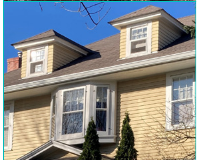
Storm windows such as these are recommended as they match the color of the historic window, and the division line matches the sash line of the historic window. City of Birmingham, photo by KDG, 2022.
