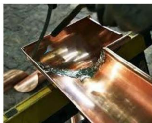
Copper Gutter Soldering Repair
