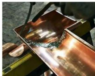
Copper Gutter Soldering Repair
