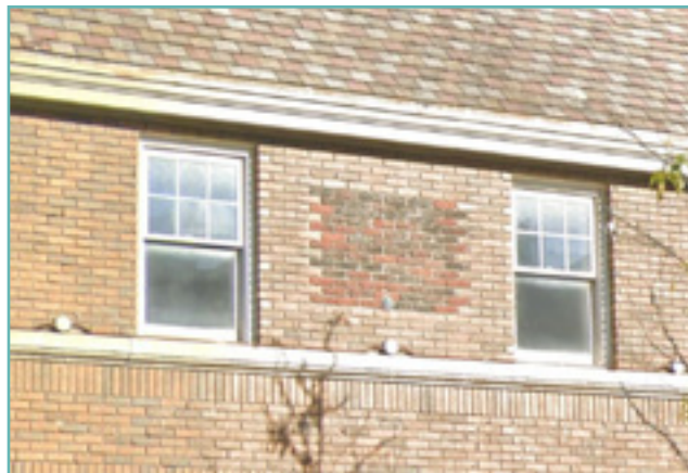
Patching historic brick with modern brick of a different color or texture on a highly visible elevation is not recommended. City of Birmingham, photo by KDG, 2022.
