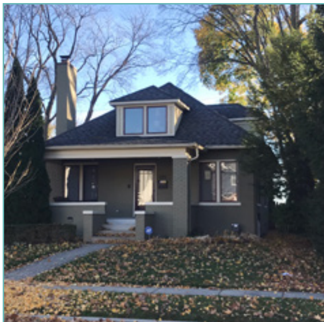
If circumstances require that modern window replacements are used, it is recommended that replacement windows match the historic windows as closely as possible. The replacement windows shown above would not be recommended as they are fixed sash windows without muntins, which do not match the historic 3-over-1 windows that were originally present. City of Birmingham, photo by KDG, 2022.
