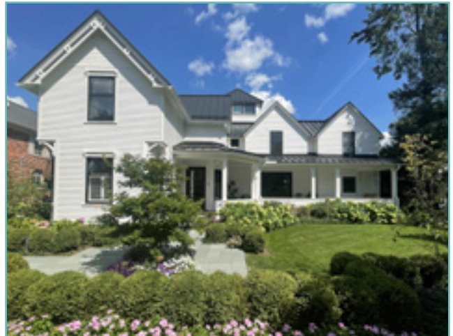
Installation of a standing seam metal roof is not recommended on historic houses where a metal roof did not exist historically. City of Birmingham, photo by KDG, 2022.
