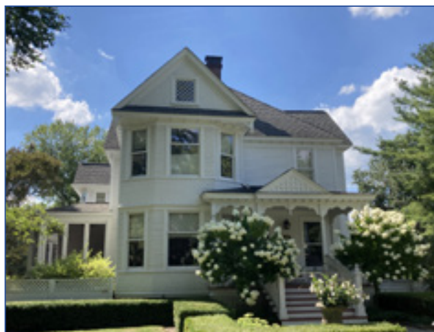
The hipped roof with lower cross gables, mixture of wood shingles and weatherboard, large porch, bay window, and irregular shape are characteristic of the Queen Anne style. City of Birmingham, photo by KDG, 2022.
