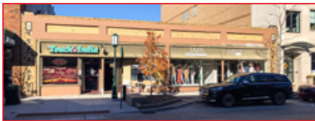
Commercial buildings typically have flat roofs that are obscured by masonry parapets, shielding the roof from view. City of Birmingham, photo by KDG, 2022.
