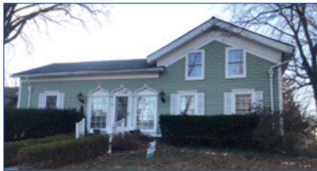
The Daniels House is an example of the Greek Revival style with its prominent entablature, 6-over-6 windows, and shallow gable roof. The ogee arches near the center of the building would have once been open, accessing a loggia. The Upright and Wing form is characteristic of Folk architecture in southeastern Michigan. City of Birmingham, photo by KDG, 2022.
