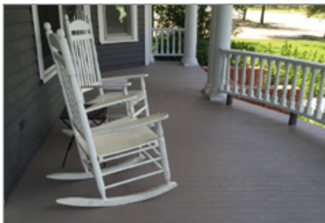
Selecting historically appropriate colors, dimensions, and textures can make the use of composite decking a viable alternative if repair or replacement of a historic wood porch or patio is not possible. Photo courtesy of Buck the Builder.
