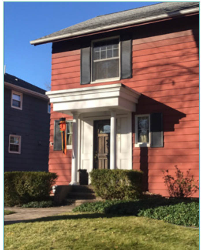
Replacement of the original porch columns is acceptable if the original columns are deteriorated beyond repair; however, it is recommended that replacement columns match the originals in terms of dimensions and detail. In the example above, the replacement columns are too slender for the porch. City of Birmingham, photo by KDG, 2022.
