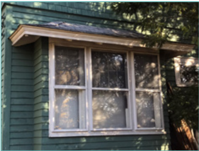
Maintaining the paint of exterior wood materials is a key component of historic house maintenance. Here, the exterior wood cladding, wood window trim wood windows, and storm windows require basic maintenance to continue functioning properly. City of Birmingham, photos by KDG, 2022.
