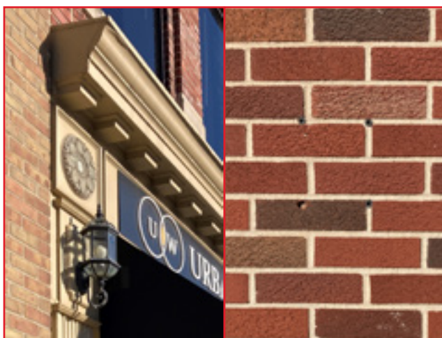
Historically appropriate lighting is shown at the left. At right shows where previous light fixtures were attached to the exterior. It is not recommended that historic material, such as the brick, be damaged when installing lighting. Lighting should be affixed at the mortar joints, City of Birmingham, photo by KDG, 2022.
