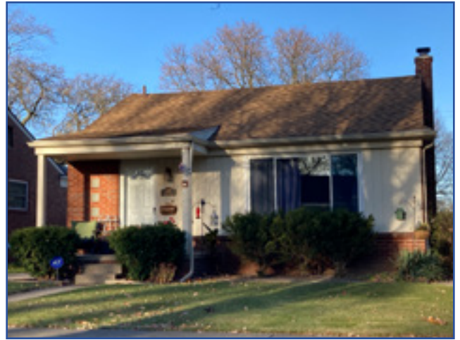
This small, Ranch style house has a side gable roof, large picture window, and cladding includes brick veneer and siding. City of Birmingham, photo by KDG, 2022.
