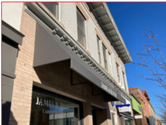
Historic awnings were generally triangularly shaped and extended outward at the base to shelter the façade. An awning may not have existed on this building historically, but this type of modern awning is acceptable. City of Birmingham, photo by KDG, 2022.
