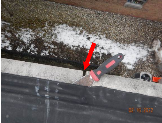
13. View of typical unadhered edge of the EPDM membrane covering the termination-bar. Note, open head joint in the stone coping (arrow).
