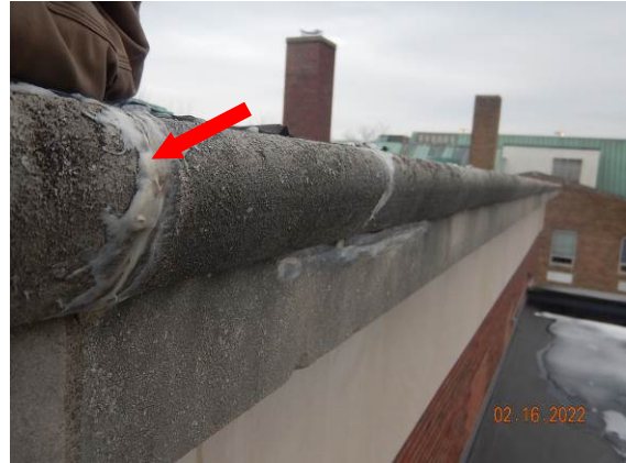
14. View of typical epoxy repair to cracked/spalled bullnose of stone coping. Note, epoxy has been used to fill some of the head joints of the coping (arrow).
