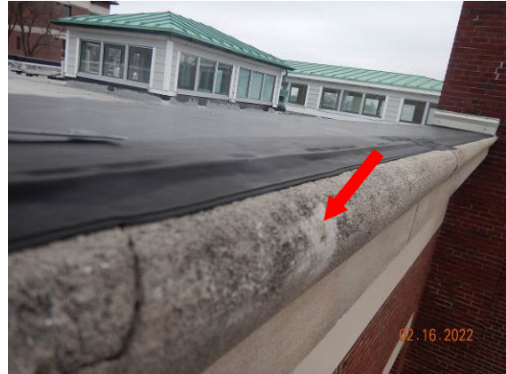
20. View of stone patch used at bullnose repair. Note, crack in Photos 19 and 20 is the same crack.
