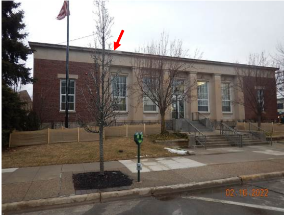
1. Overview of the main entrance on the south elevation of The Surnow Building. A section of precast stone has spalled off the outer edge of the coping (arrow).
