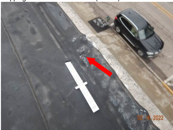
11. View of typical punctures and/or holes in the EPDM stripping membrane that covers the termination-bar.
