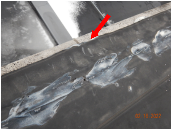
17. The epoxy used for repair of cracked/spalled coping bullnose has been applied over holes in the EPDM stripping membrane and used to adhere the outer edge of the membrane.
