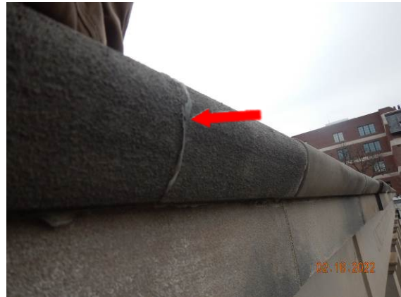
4. View of bullnose on outer edge of stone coping. Note location of previous epoxy repair to crack (arrow).
