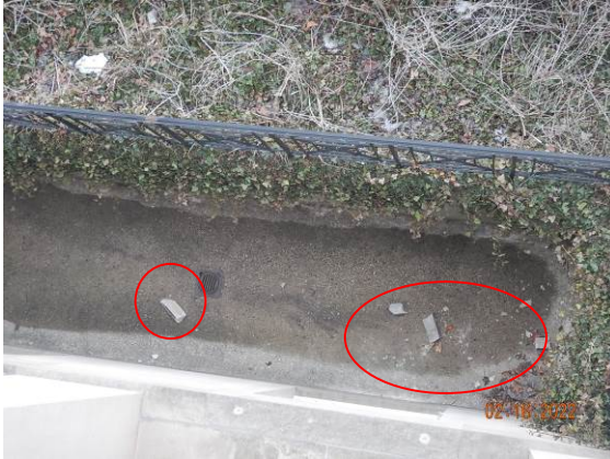
7. View of stone pieces of spall coping bullnose in window well.
