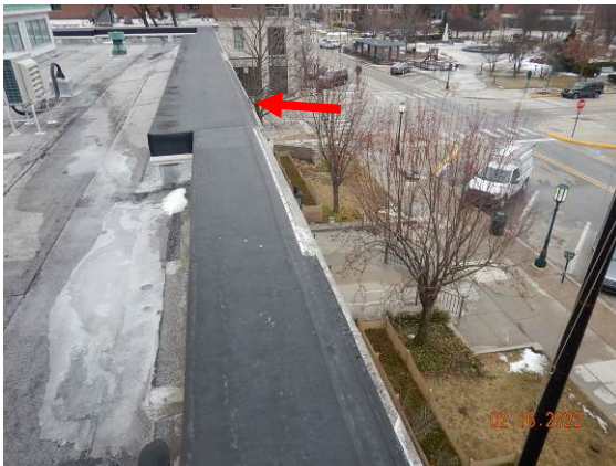
5. Overview of location of spalled and missing bullnose on south parapet coping (arrow).
