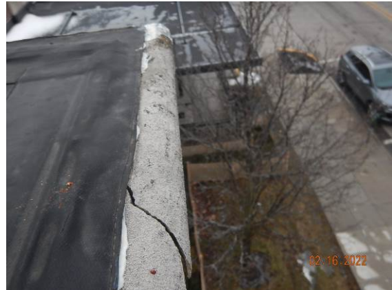
16. Additional cracking has occurred adjacent to some of the epoxy repairs to the coping bullnose.
