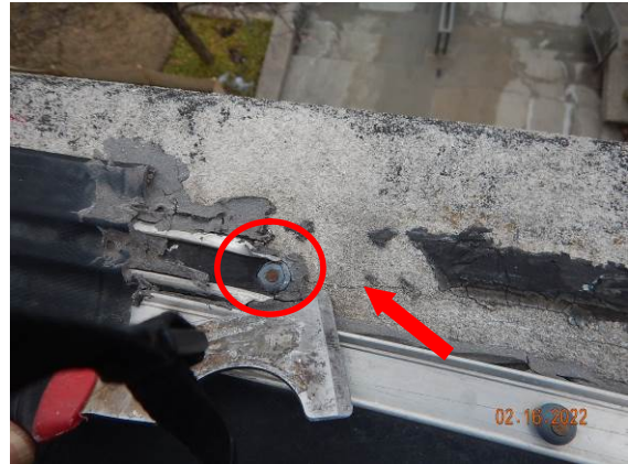
22. Closer view of stone coping crack originating at an exposed wedge anchor along bullnose on the south parapet. Note, portions of the termination-bar appear to have been removed in conjunction with the removal of the EPDM stripping membrane (circle).
