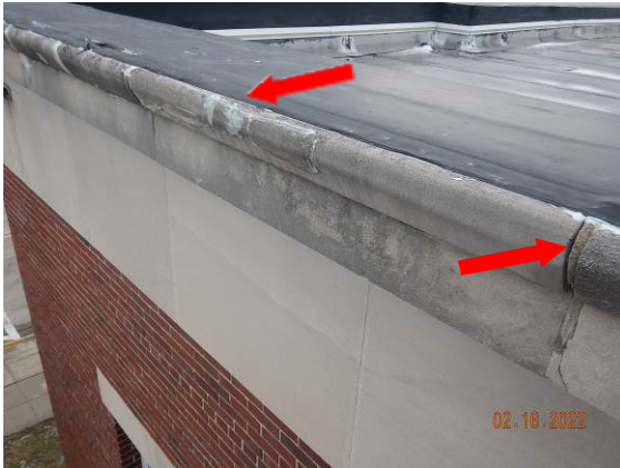
15. Overview of epoxy repair to cracked/spalled bullnose on stone coping. Note open head joint at coping bullnose.
