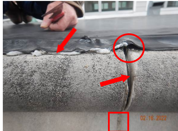
18. View of typical open head joint at bullnose of stone coping. The mortar appears to have been mechanically removed. Note epoxy along edge of EPDM membrane with opening (circle) and that the mortar was not removed below the bullnose (square).
