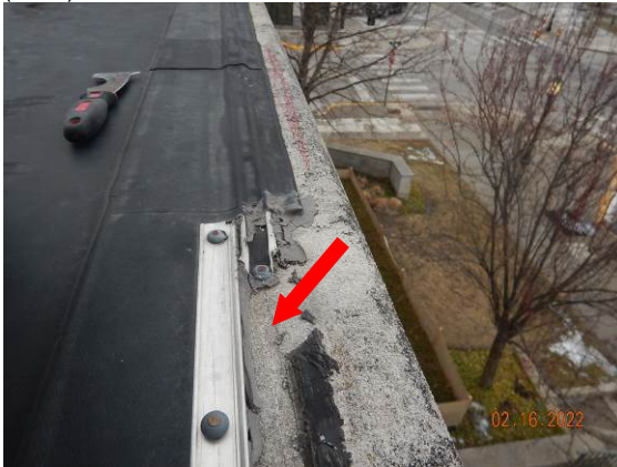
21. View stone coping crack originating at an exposed wedge anchor along bullnose on the south parapet. The section of bullnose appears loose and is a fall hazard.
