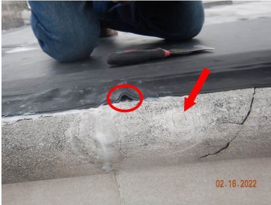
19. View of stone patch used at bullnose repair. Note, epoxy was used to adhere the outer edge of the EPDM stripping membrane, although, there is still an opening (circle).
