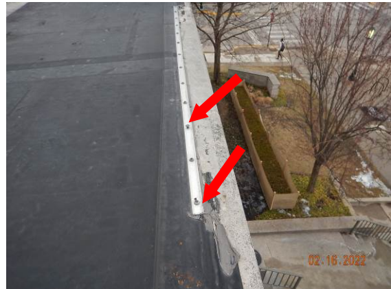
10. Closer view of an exposed portion of EPDM termination. Note, some of the wedge anchors used to secure the termination-bar are working out (arrows).
