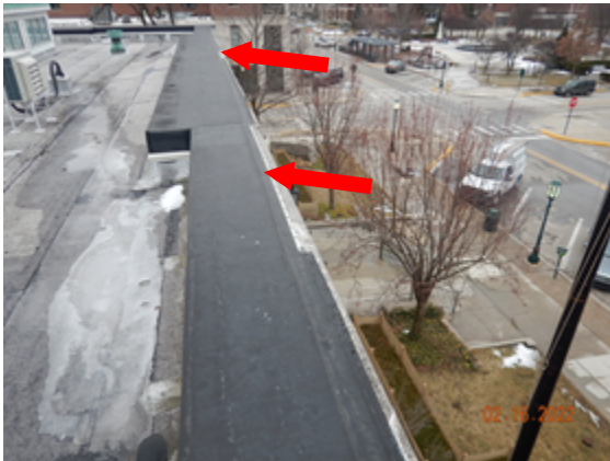
9. EPDM membrane installed atop the stone coping is terminated along the outer edge of the coping with termination-bar and lead wedge anchors. Note, at most locations' termination-bar is covered by EPDM stripping. There are two locations along the south parapet where the stripping membrane is removed (arrows).
