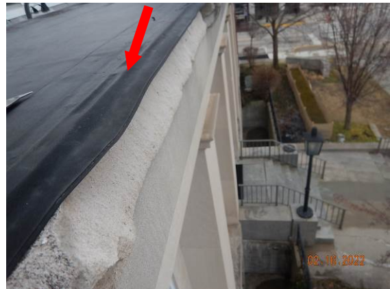
6. Closer view of spalled and missing bullnose on south parapet coping. Note, spall is at location of termination-bar (arrow).
