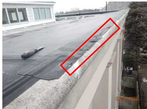
12. View of multiple open ridges at the out edge of the EPDM membrane covering the termination-bar.
