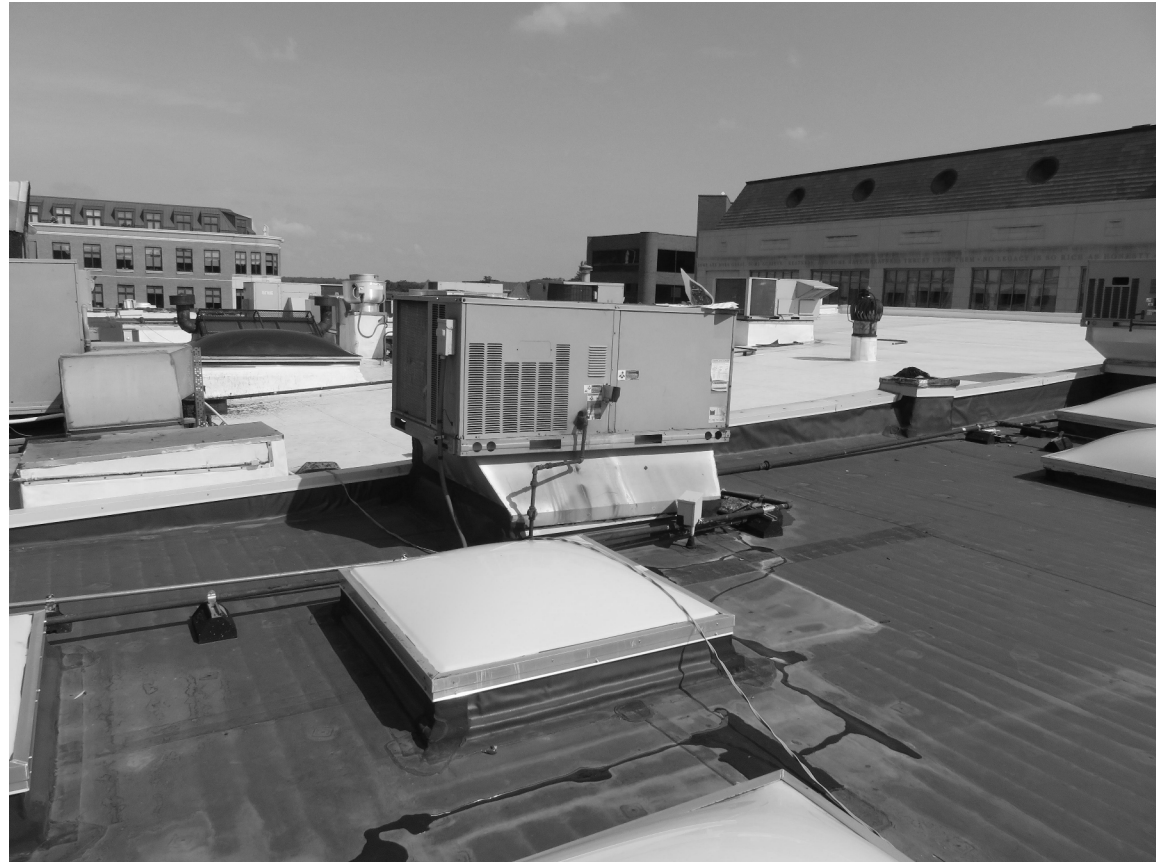
EXISTING RTU & RTU'S IN VICINITY OF SPACE
