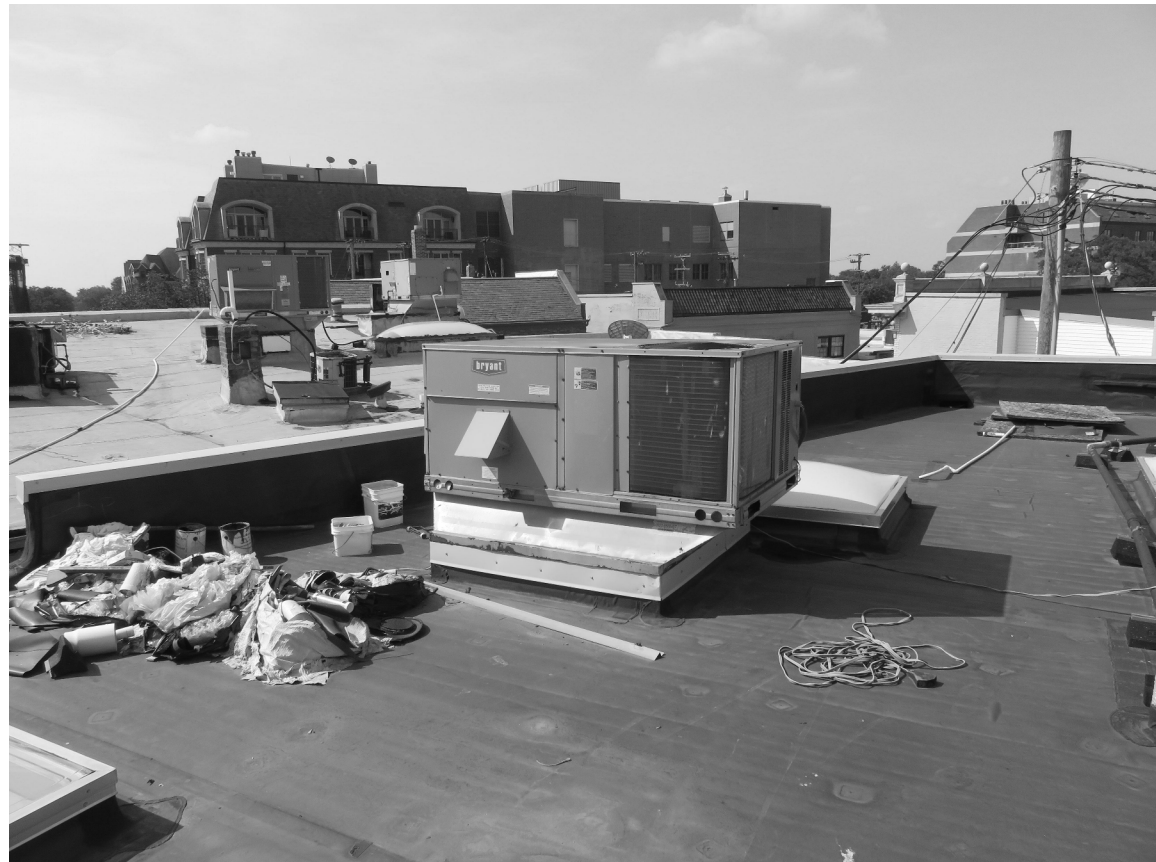
EXISTING RTU & RTU'S IN VICINITY OF SPACE
