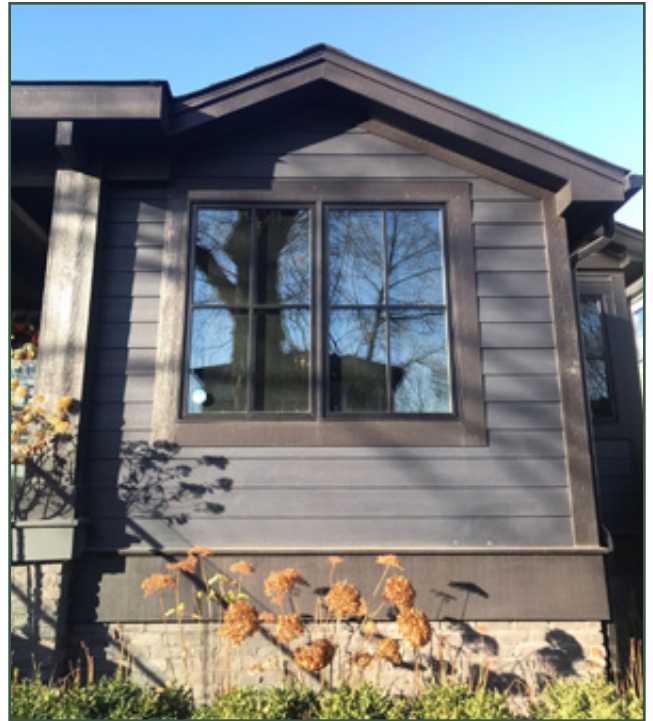
Although this modern replacement siding has a different finish than historic wood siding, it mimics the texture of wood and is a viable replacement for wood cladding too deteriorated to repair or preserve.
