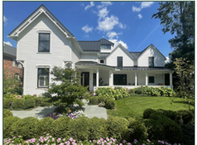
Installation of a standing seam metal roof is not recommended on historic houses where a metal roof did not exist historically.
