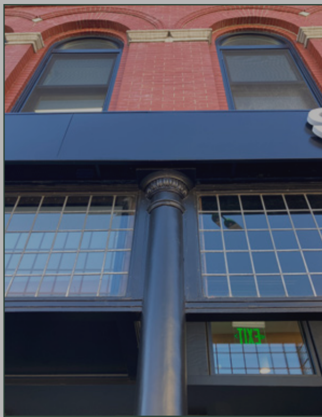
The metal elements of this storefront have been adequately maintained
