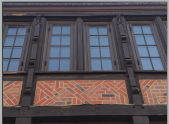
Maintenance and repair of original wood exterior details is key. The wood in the image above requires some repair from water damage and repainting.
