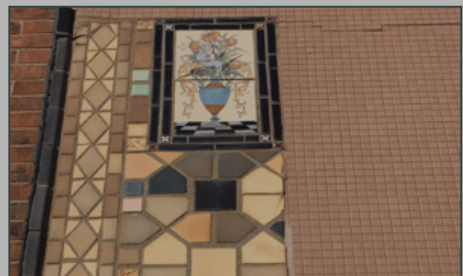
The replacement of the historic tile on the left side of the image with modern tile on the right is not recommended
