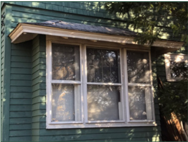
Maintaining the paint of exterior wood materials is a key component of historic house maintenance. Here, the exterior wood cladding, wood window trim wood windows, and storm windows require basic maintenance to continue functioning properly.
