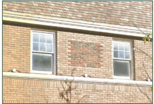
Patching historic brick with modern brick of a different color or texture on a highly visible elevation is not recommended.
