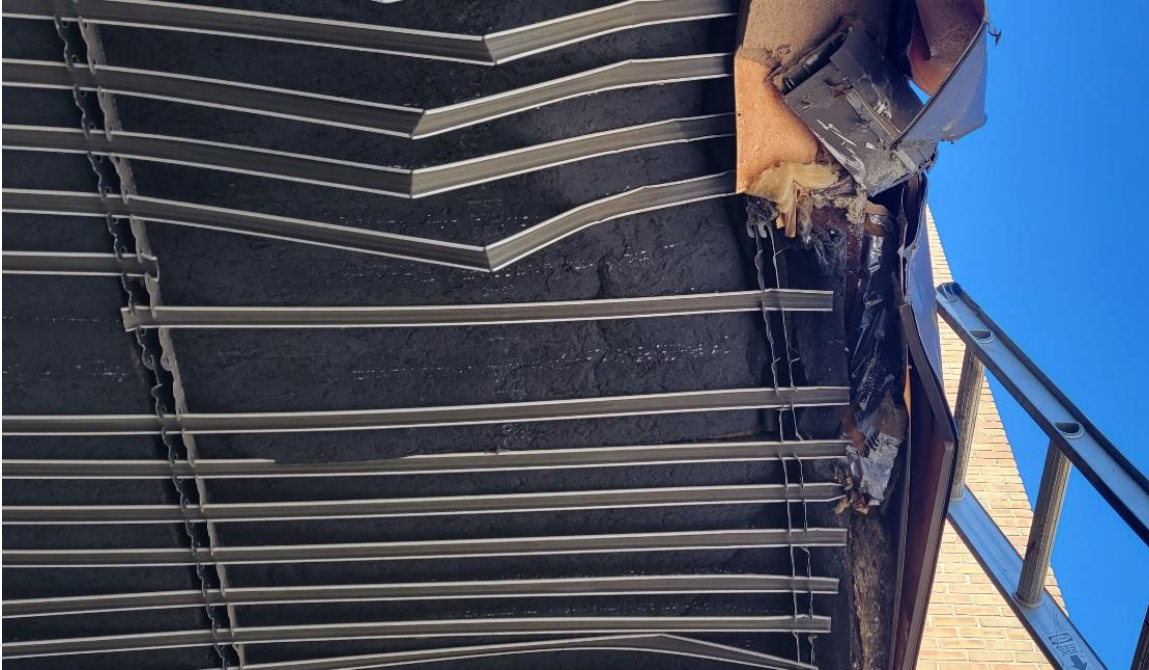
Figure 7. Damaged hat channel ceiling panel system near impact area.
