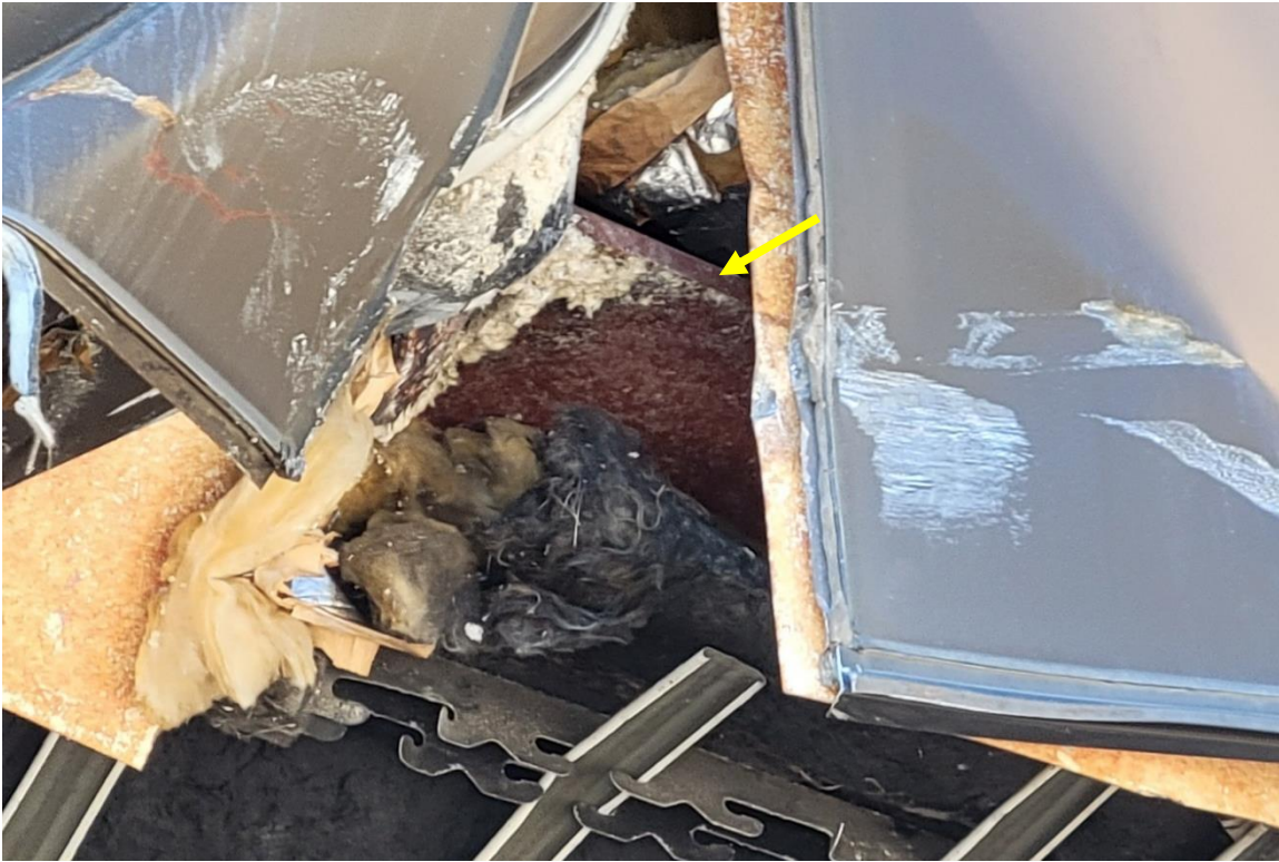
Figure 5. Exposed bottom flange of the structural steel beam at the impact area.
