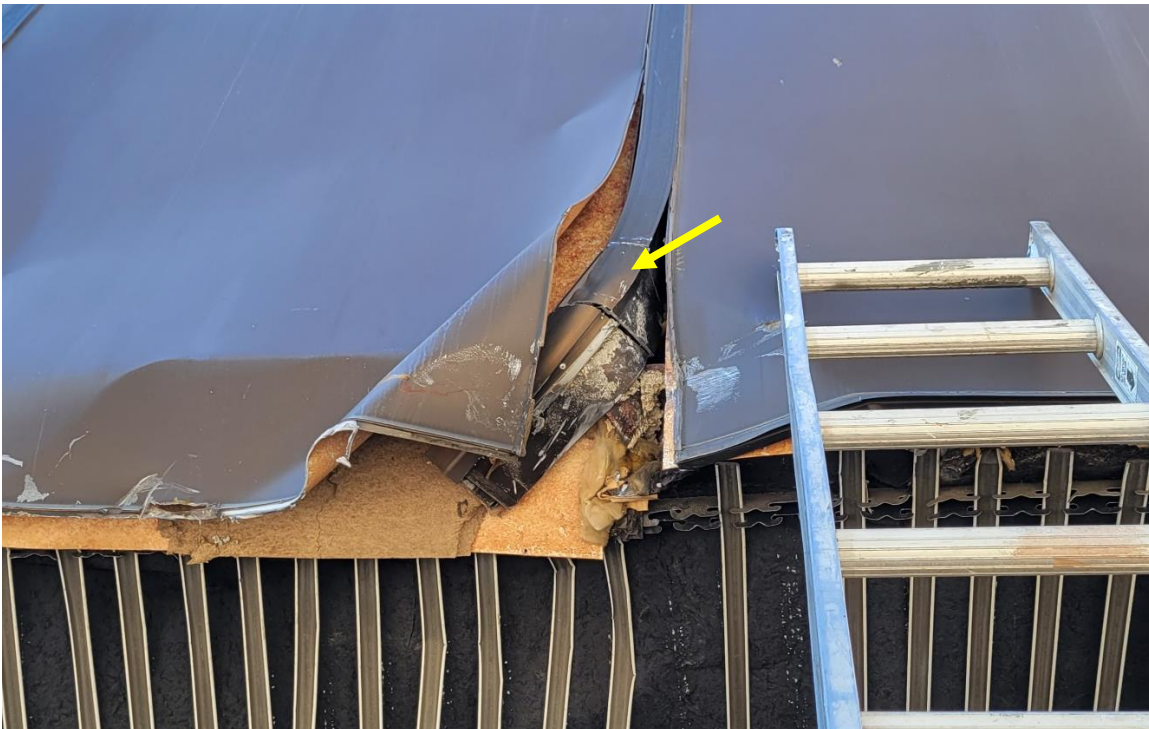
Figure 4. Damaged architectural cladding and mullion (yellow arrow).
