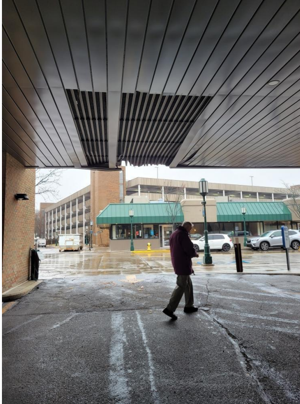
Figure 1. Overview of impact damage to ceiling panel prior to WJE's site visit (photograph provided by CBRE).
