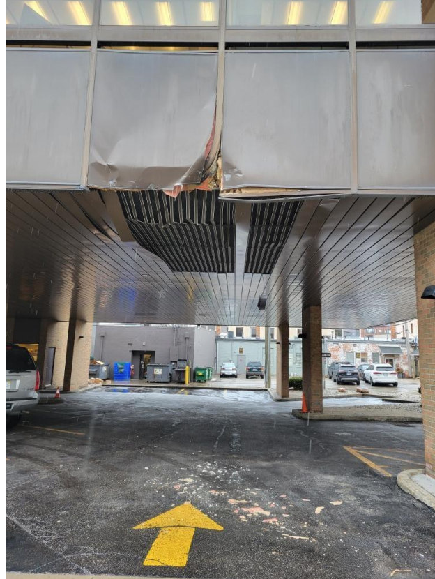
Figure 2. Overview of impact damage to north facade prior to WJE's site visit (photograph provided by CBRE).
