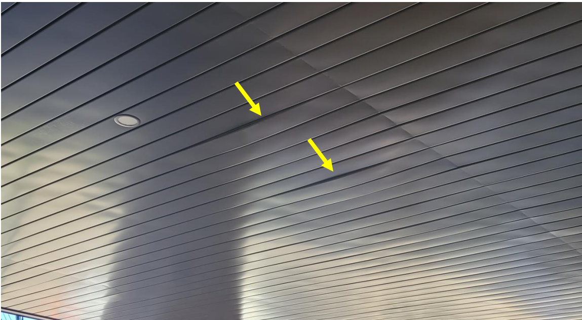
Figure 8. Ceiling panels on the south side of parking level displaced downward.
