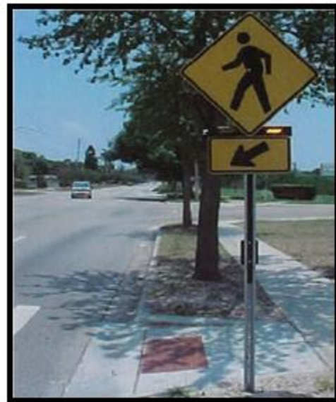
Figure 9: Example of RRFB with W11-2 sign and W16-7p plaque at unsignalized crosswalk. [Photo courtesy of City of St. Petersburg, Florida]
