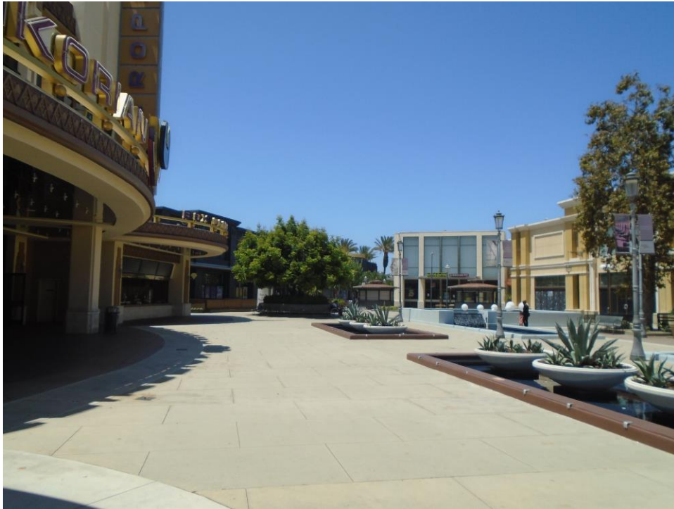
Figure 7. Southern Addition: overview of open-air pedestrian walkway between buildings, view to west (DSC03505)
