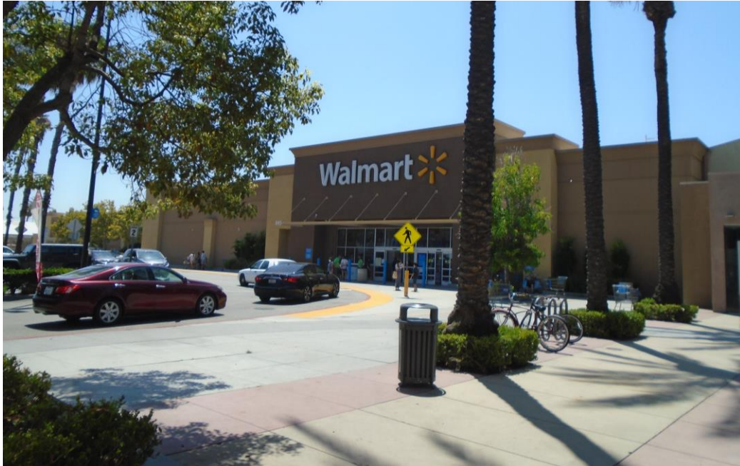
Figure 18. Eastern Addition: north (main) elevation, view to south (DSC03427)
