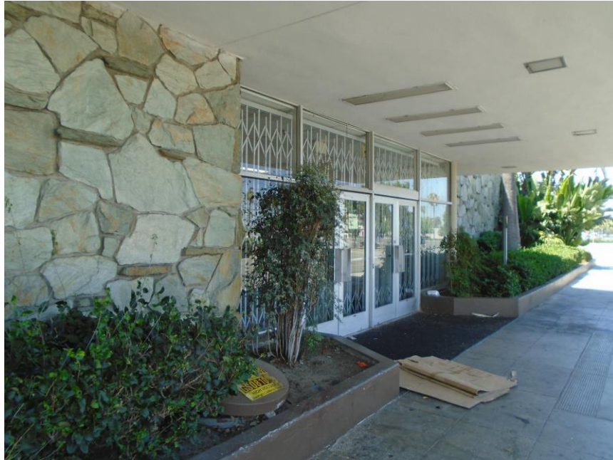
Figure 3. Sears: north elevation entrance, view to southwest (DSC03268)
