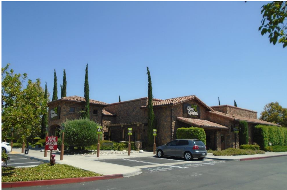
Figure 19. Northern Detached Building: example of one of the four northern buildings, view to northeast, constructed in 2004 (DSC03438)
