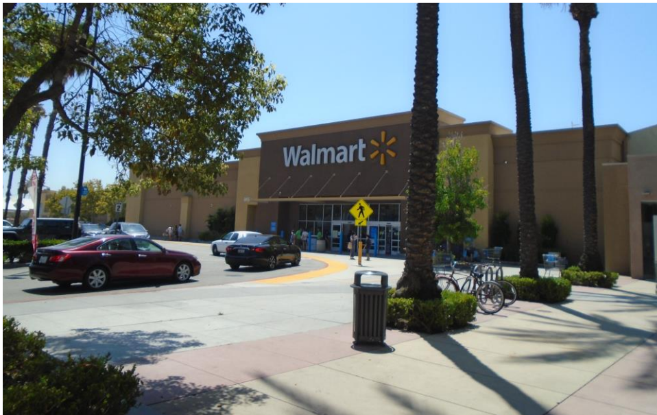
Figure 8. Eastern Addition: north (main) elevation, view to south (DSC03427)
