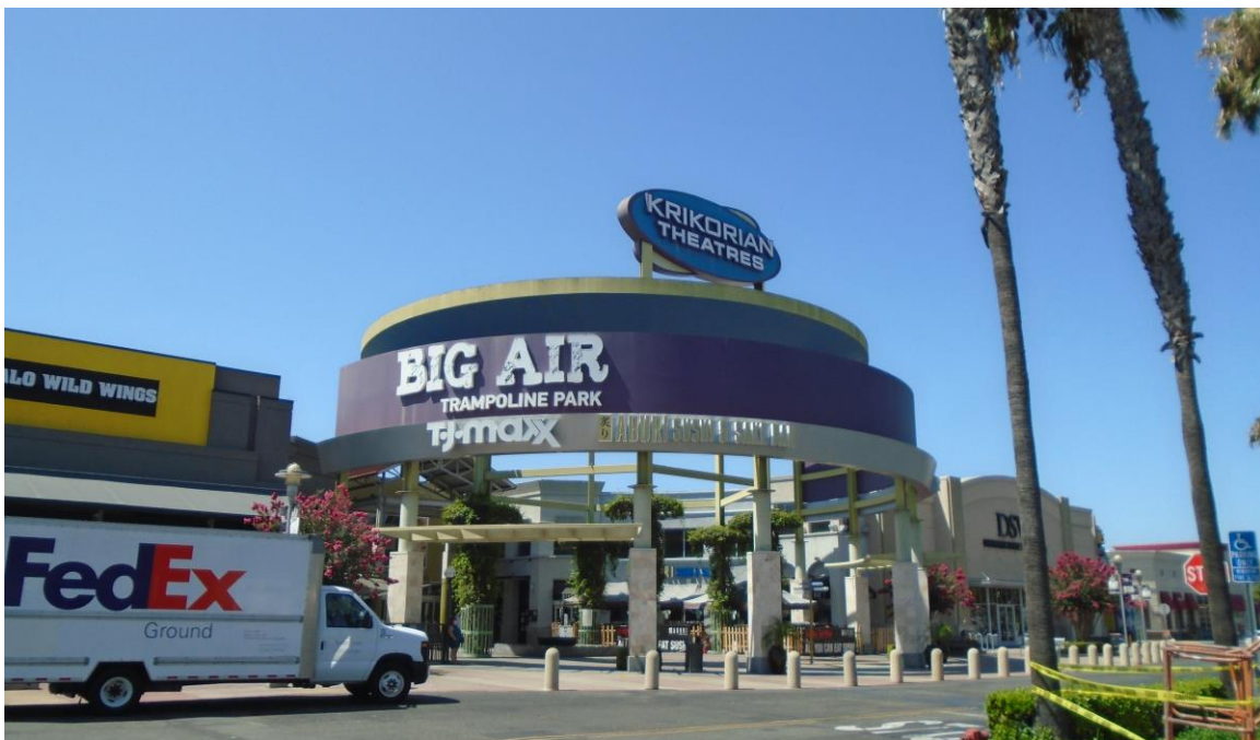
Figure 6. Central Mall Addition: main entrance, main (north) elevation, view to south (DSC03202)
