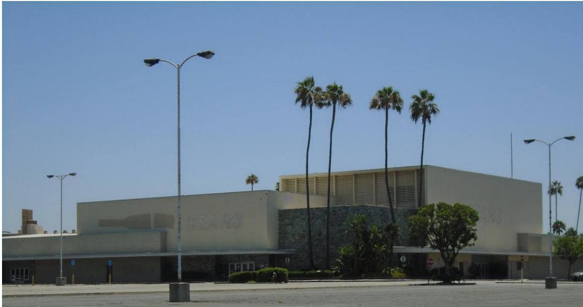
Figure 12. Sears: north and west elevation, view to southeast (DSC03447)
