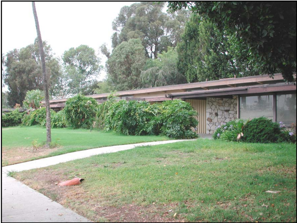
Plate III. Top: Northwesterly view of the recreational wing of the Recreational/Administrative building. Bottom: Northwesterly view of administrative wing of the Recreational/Administrative building.
