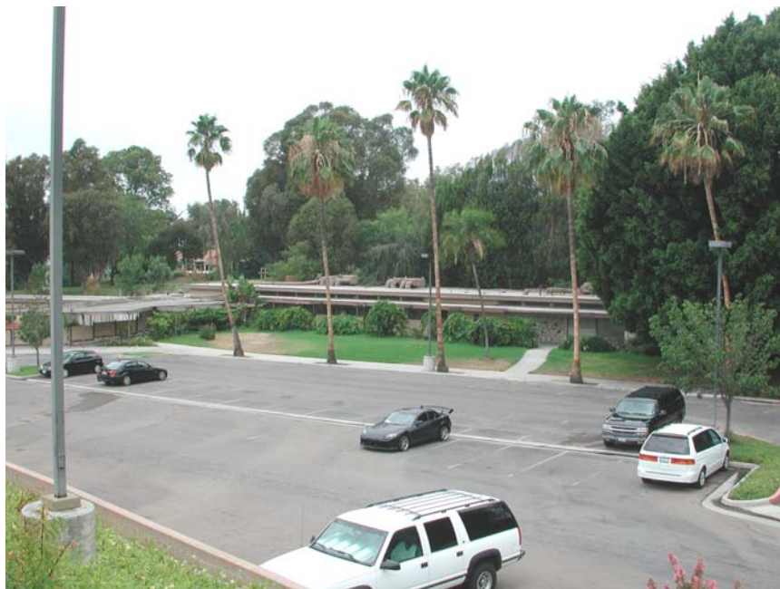
Northwesterly view of Administration (Facilities Management) Building.
