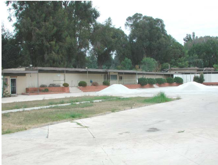
Northeasterly view of recreational building (former Tennis office, showers, locker rooms, and snack bar). Former pool area in foreground.
