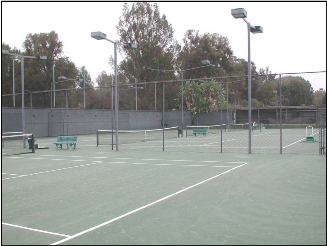
Plate I. Top: Westerly view across west tip of Zone A. Bottom: Northeasterly view through large tennis courts slated for demolition in Zone A.
