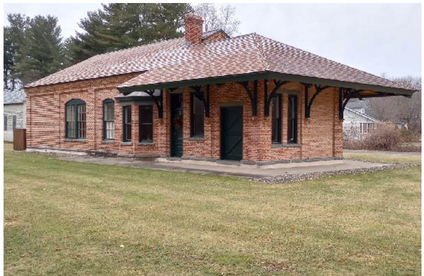
The restored trolley station in North Chatham was in use 1900 - 1929 (D. Hegeman)
