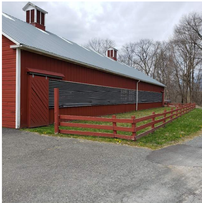
PHOTO 14: EAST SIDE OF BARN 4 EXTERIOR
