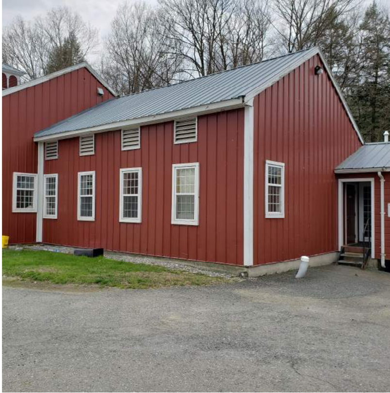
PHOTO 11: WEST SIDE OF BARN 2 EXTERIOR LIGHTING
