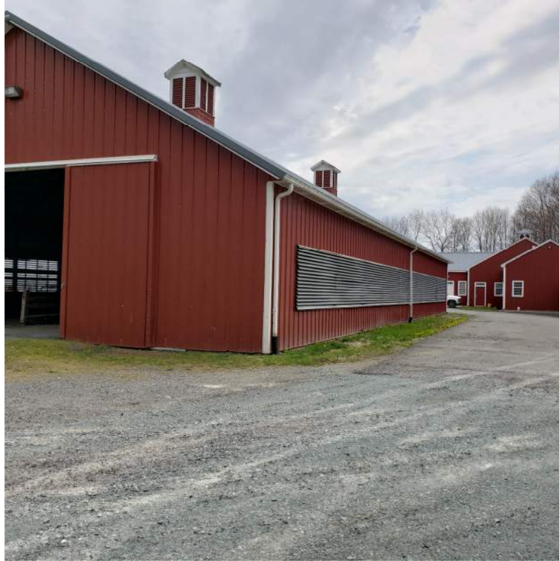
PHOTO 15: WEST SIDE OF BARN 4 EXTERIOR
