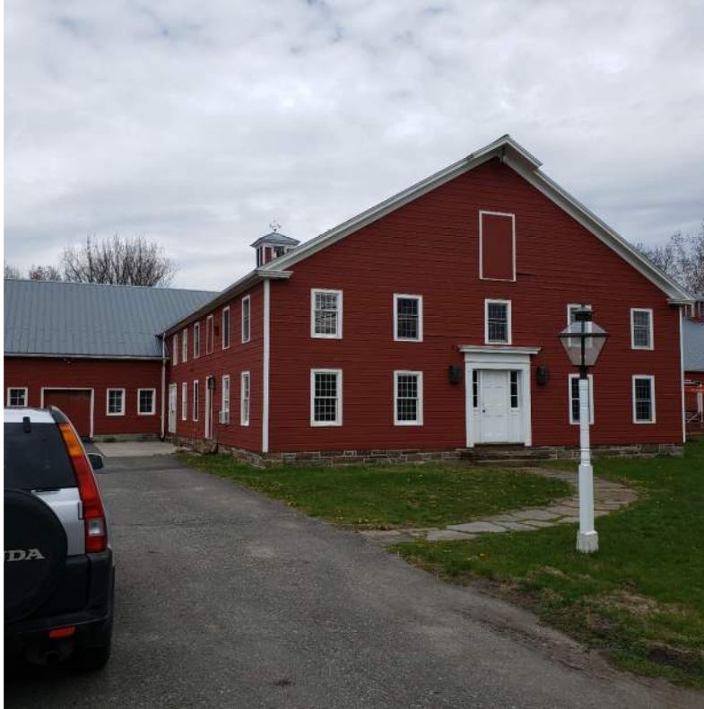
PHOTO 1: MAIN ENTRANCE (SOUTH SIDE) OF BARN 1 EXTERIOR LIGHTING
