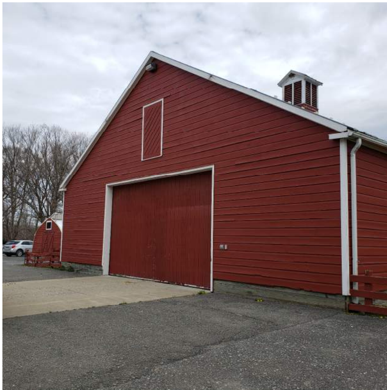
PHOTO 4: WEST SIDE OF BARN 1 EXTERIOR LIGHTING
