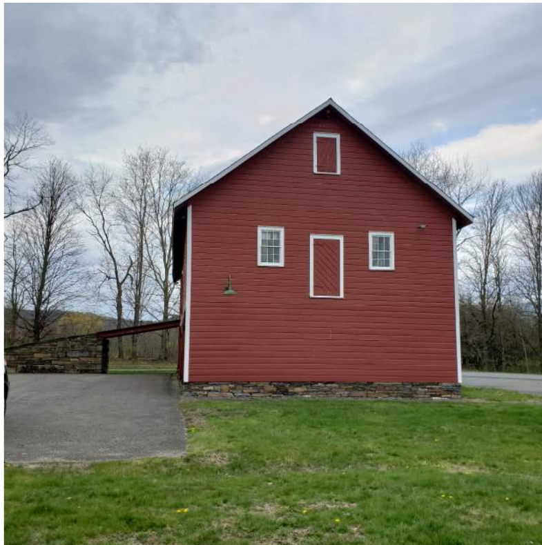
PHOTO 8: NORTH SIDE OF BARN 2 EXTERIOR LIGHTING
