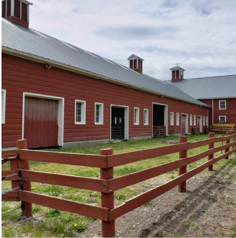
PHOTO 7: REAR (NORTH SIDE) OF BARN 1 EXTERIOR LIGHTING
