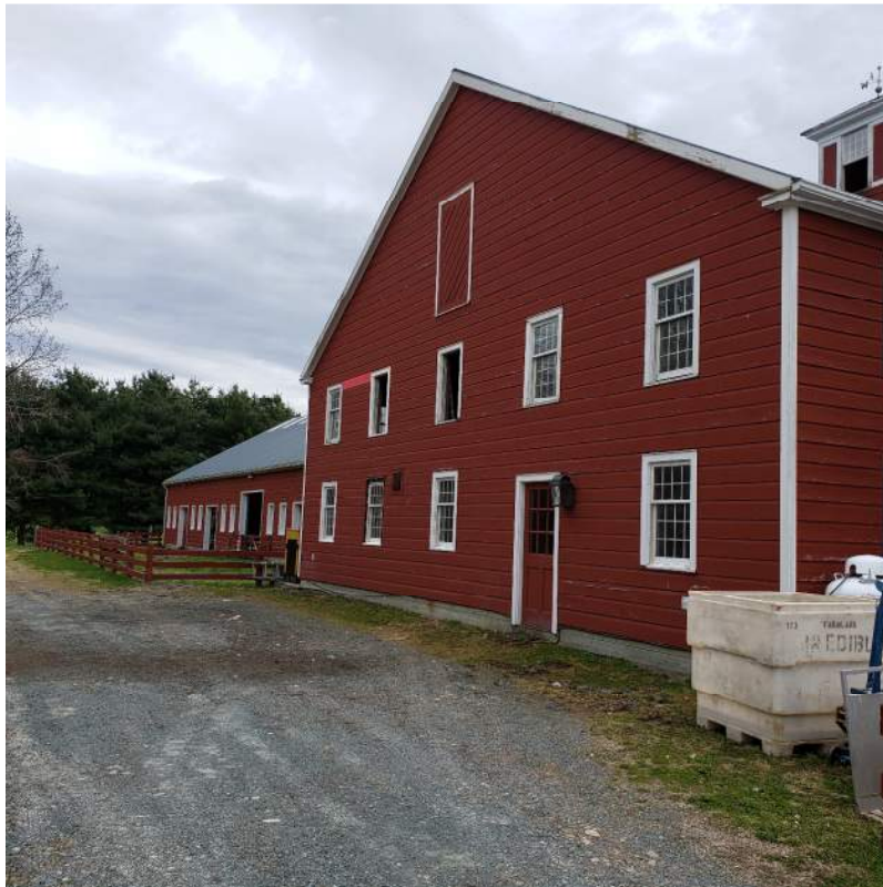
PHOTO 6: REAR (NORTH SIDE) OF BARN 1 EXTERIOR LIGHTING
