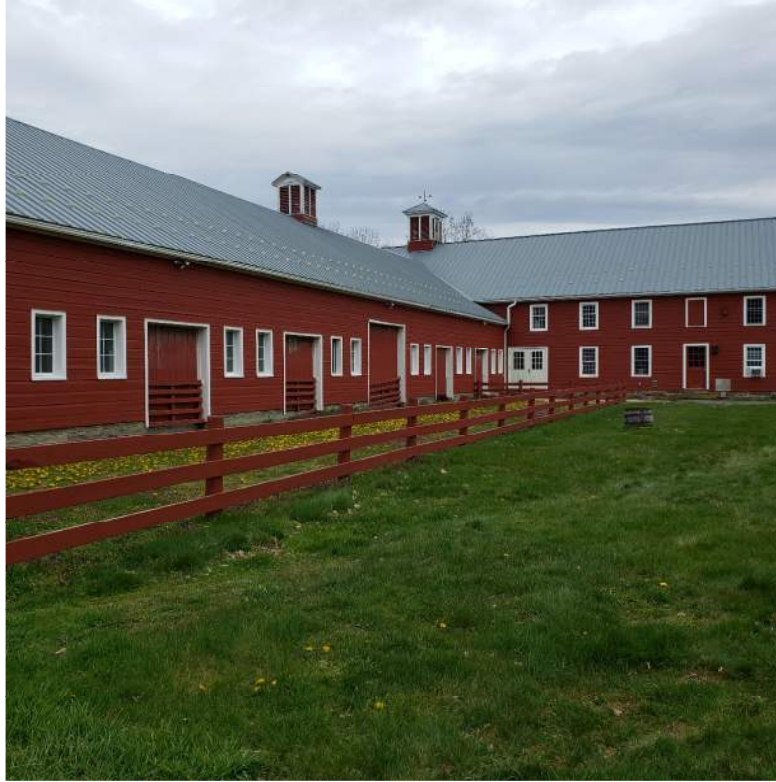
PHOTO 3: FRONT (SOUTH SIDE) OF BARN 1 EXTERIOR LIGHTING
