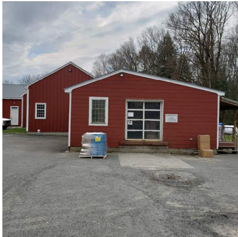
PHOTO 12: NORTH SIDE OF BARN 3 EXTERIOR LIGHTING
