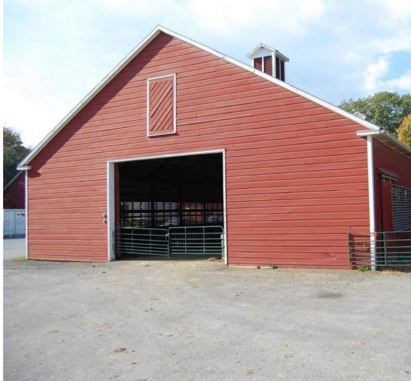
PHOTO 13: FRONT (SOUTH SIDE) OF BARN 4 EXTERIOR
