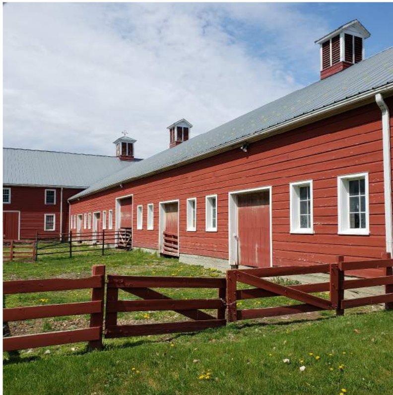
PHOTO 2: FRONT (SOUTH SIDE) OF BARN 1 EXTERIOR LIGHTING
