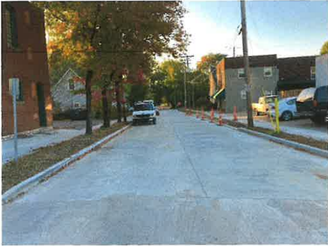
Looking southeast, aprons ready for concrete
