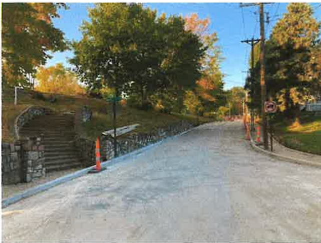
Lower portion is open. Upper portion remains closed due to a sharp turn up top. Sidewalk is ready for concrete. Upper portion should be poured next week.
