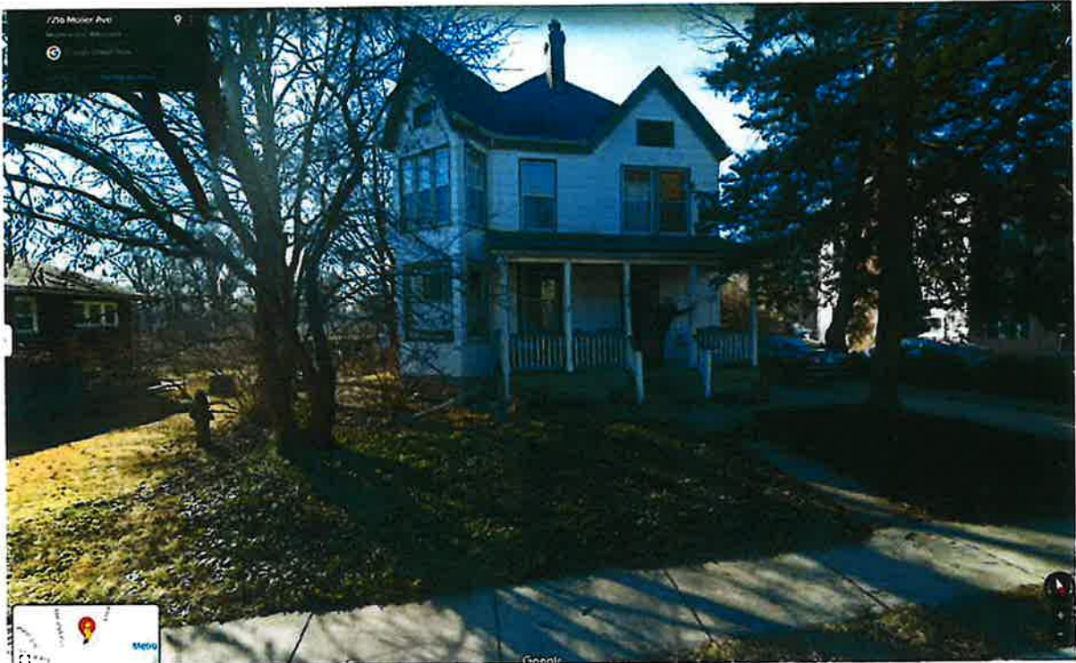
7216 Moller Avenue - House with adjacent driveway off of Moller Avenue
