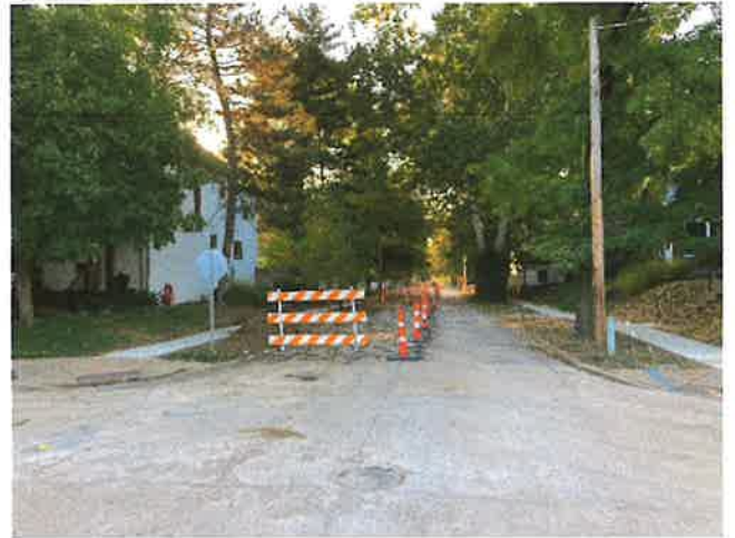
Looking southeast ready for tear out
