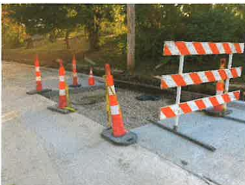
Lower portion is open. Upper portion remains closed due to a sharp turn up top. Sidewalk is ready for concrete. Upper portion should be poured next week.
