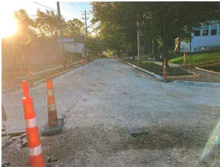
Southeast lane is open. Aprons are prepped for concrete.
