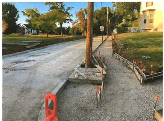
Lower portion is open. Upper portion remains closed due to a sharp turn up top. Sidewalk is ready for concrete. Upper portion should be poured next week.
