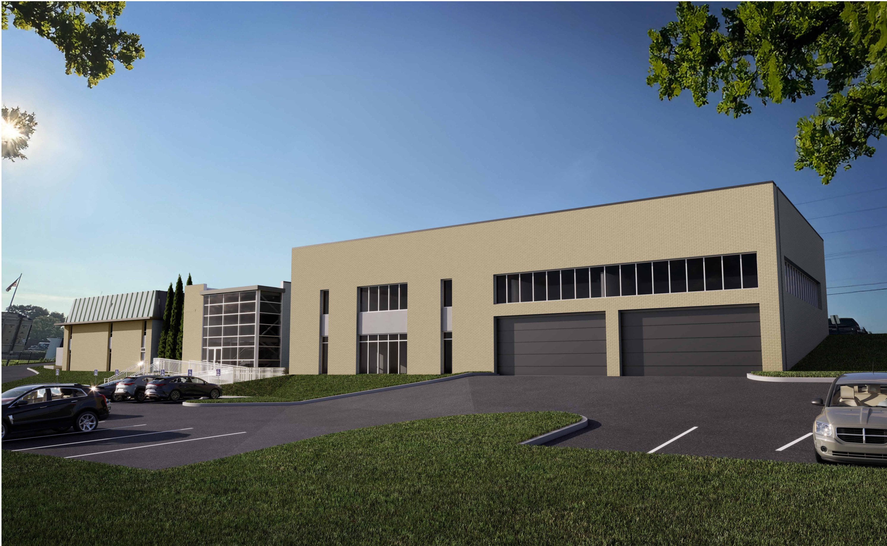
VIEW AT NORTHWEST CORNER
