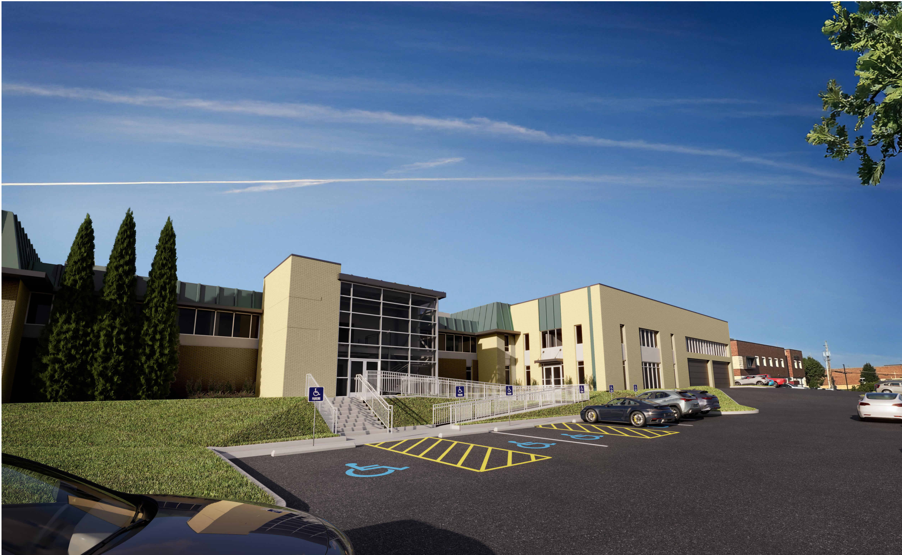
VIEW AT NORTHEAST CORNER
