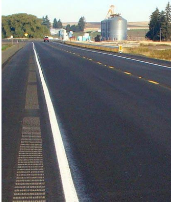
Shoulder rumble strip
