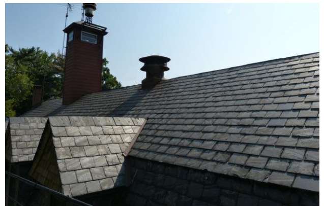
Fire Engine House 44 Roof Replacement
