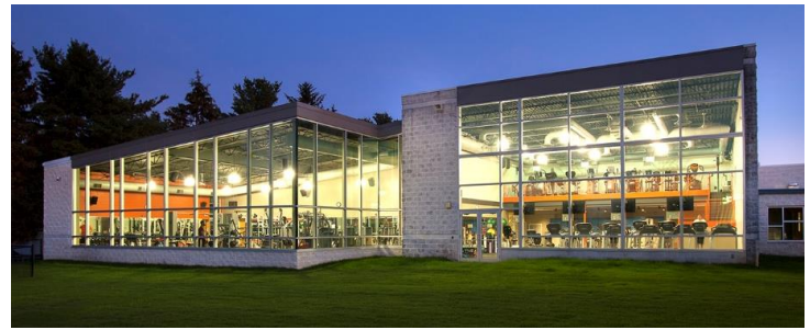
Fitness Center Addition Jewish Community Center, York, PA
