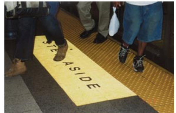
Figure 4.1c.6. The colored and textured floor strip helps everyone notice the edge of this train platform.
