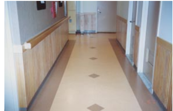
Figure 4.1c.7. To assist the wayfinding needs of those with low vision, contrasting strips were placed along the edges of the hallway and dark brown diamond shapes were imbedded in the center of the path of travel.
