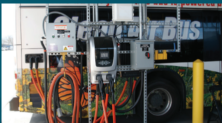
Each bus plugs into one of 18 charging stations at night, with HotStart technology to keep batteries warm in the winter.
