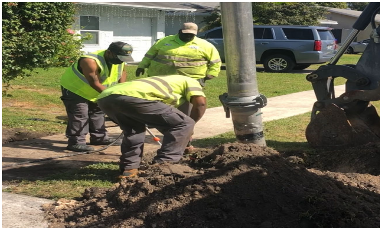
Utilities team works on meters.
