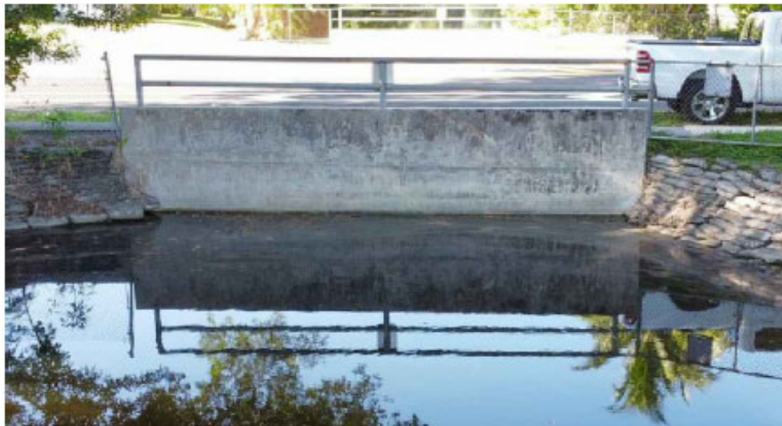
EXISTING TWIN 40-INCH CMP CULVERT HEADWALL (NORTH SIDE OF KIMBERLY BLVD)
