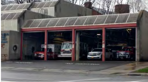
City of Oneonta Public Safety Building. Photo Credit: Oneonta Fire Department
