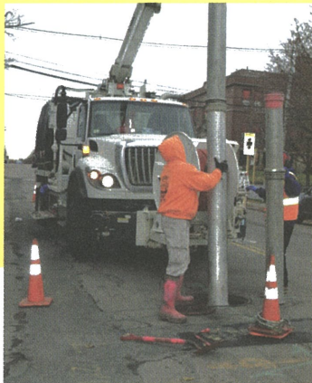
A Sewer Operations technician removes debris from a sewer.
