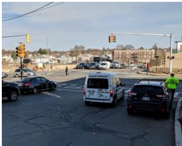
Figure 10 - Lane movement markings not provided for Beale Street eastbound
