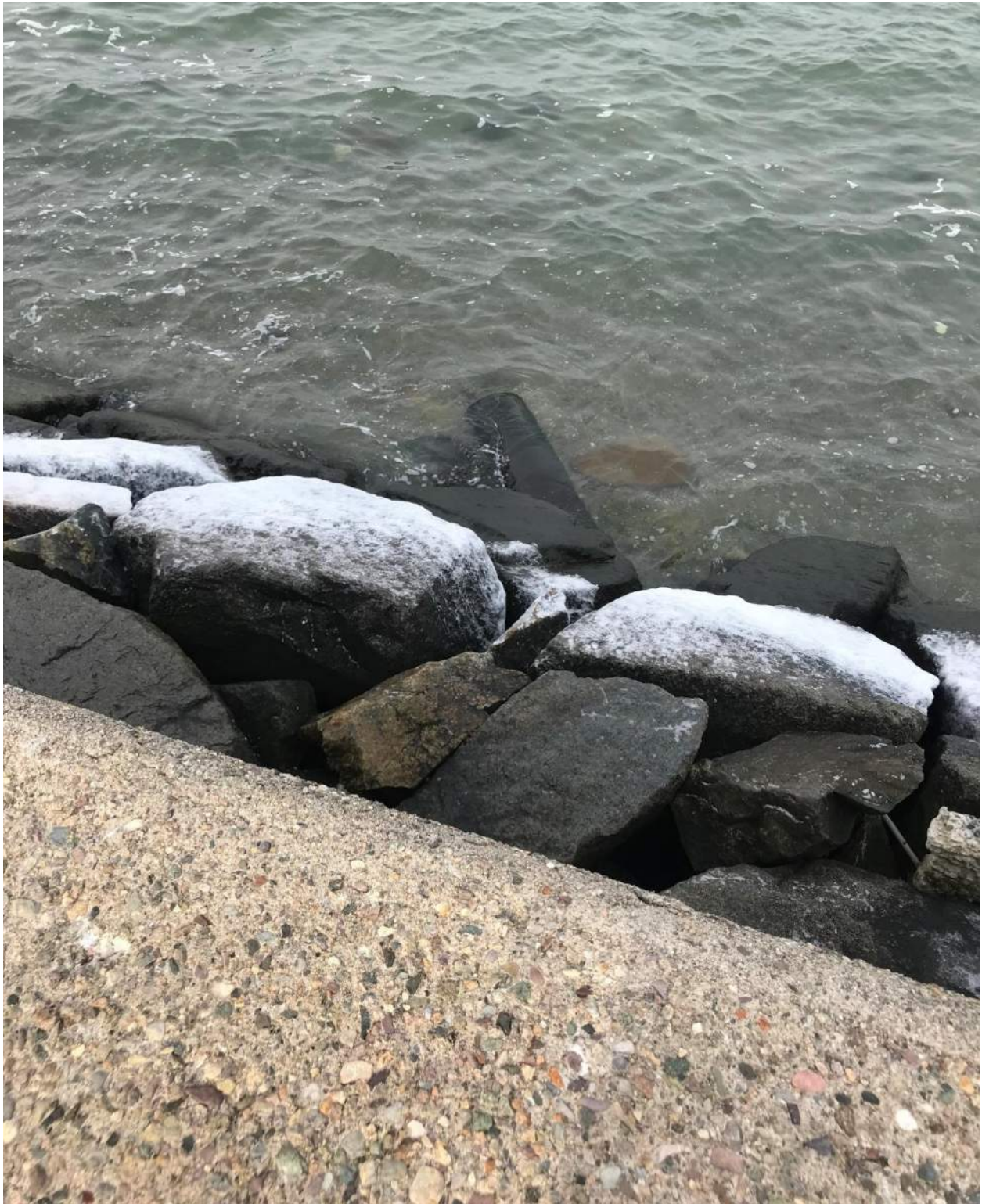
Photo 2: Looking north from the seawall at a 12-inch diameter outfall (OF-02506) near the intersection of Sea Street and Babcock Street (12/14/17).
