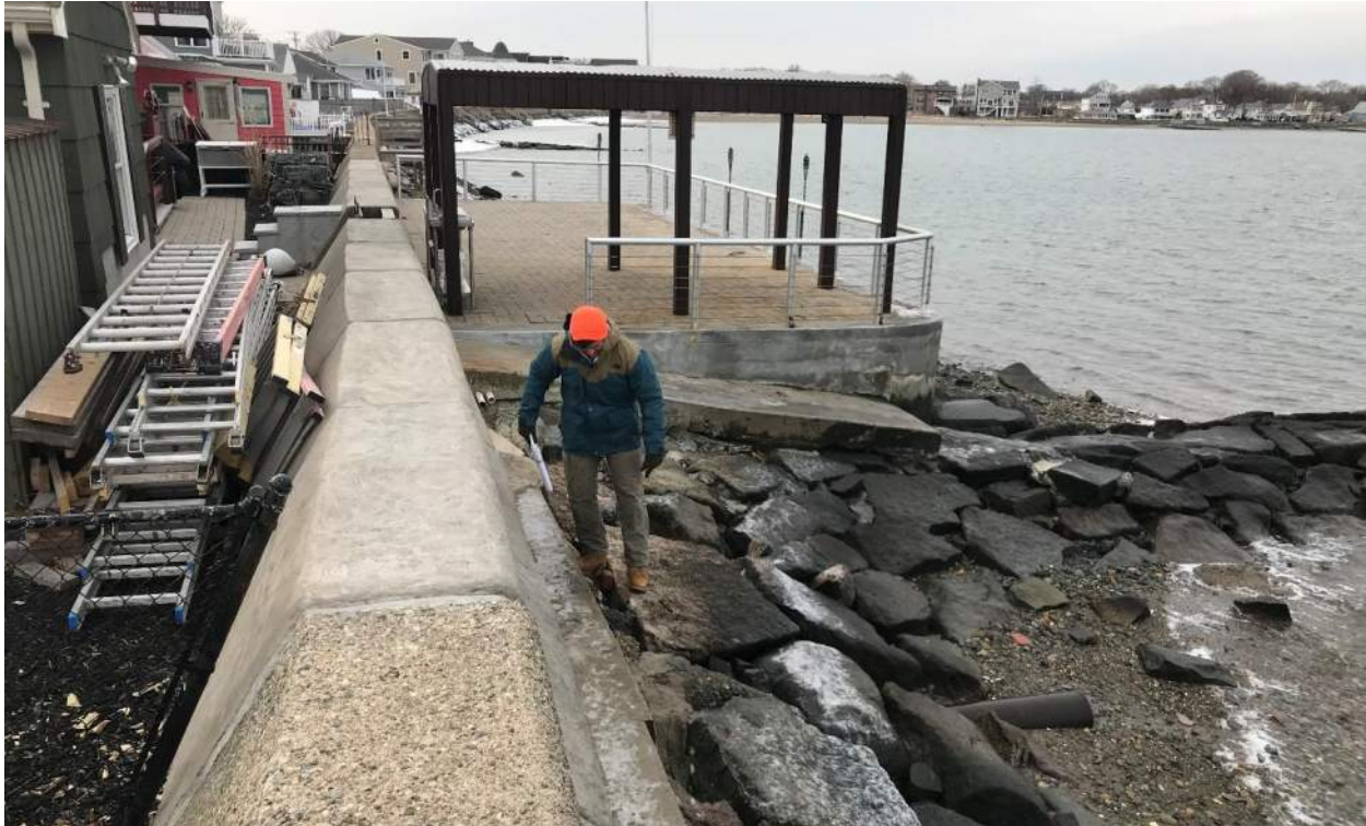
Photo 4: Looking west at a gazebo and ramp on the seaward side of precast concrete seawall, adjacent to a groin and 12-inch diameter outfall (OF-02708) near 752 Sea Street (12/14/17).
