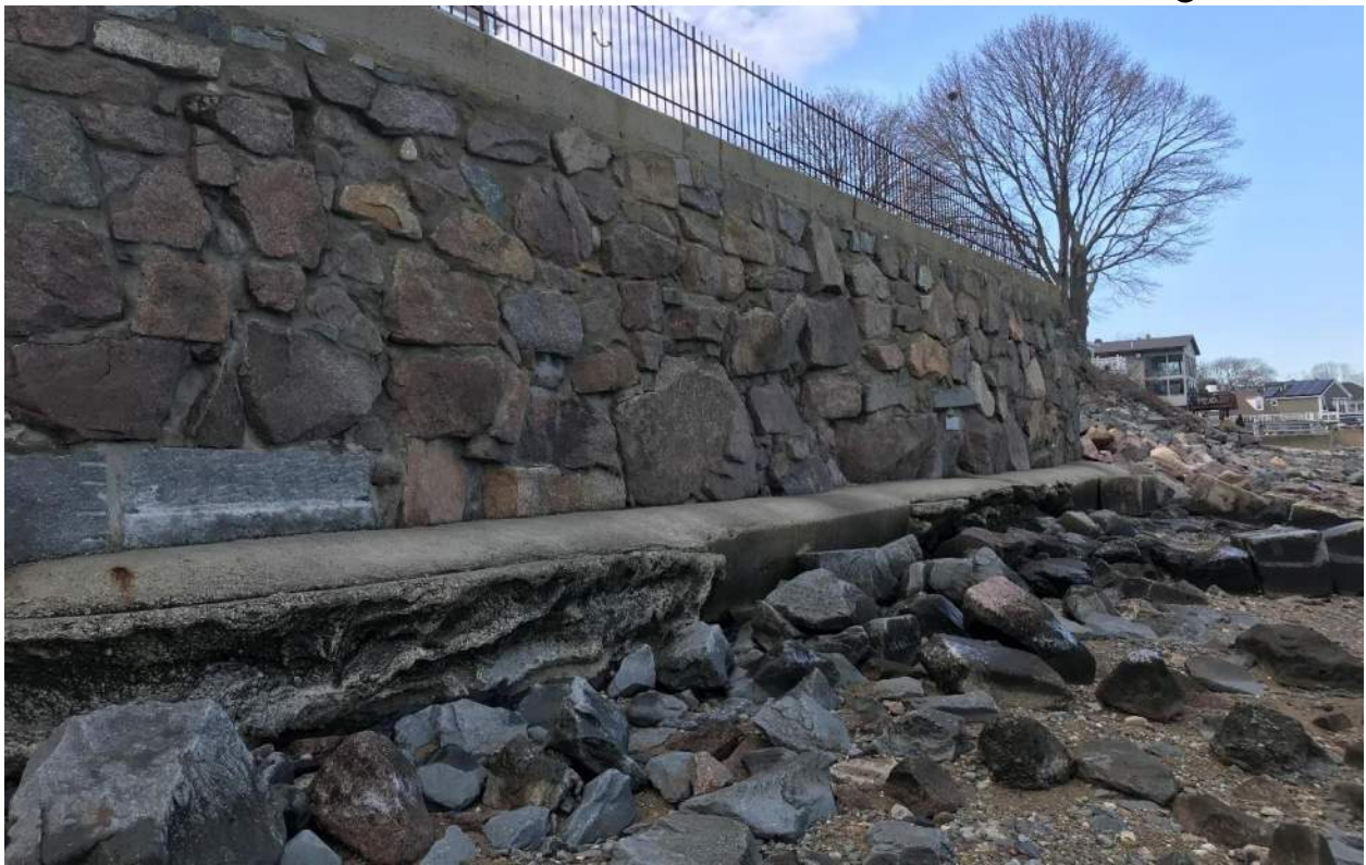
Photo 33: View of private stone and mortar wall capped with poured concrete looking south-southwest toward revetment area near 24 Norton Road (12/14/17).
