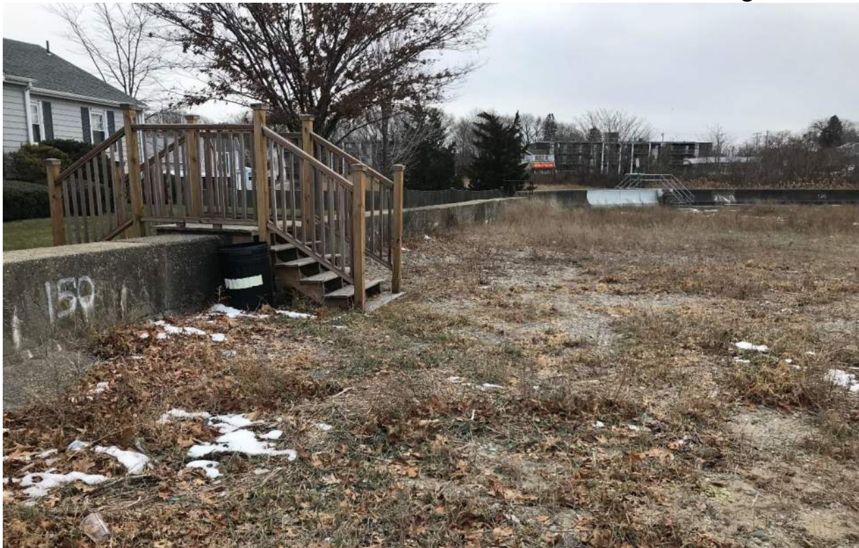
Photo 27: View looking south at cast in place concrete seawall near Norton-Terne beach area; beach area is on right, 32 Terne Road is on left side of photo (12/14/17).
