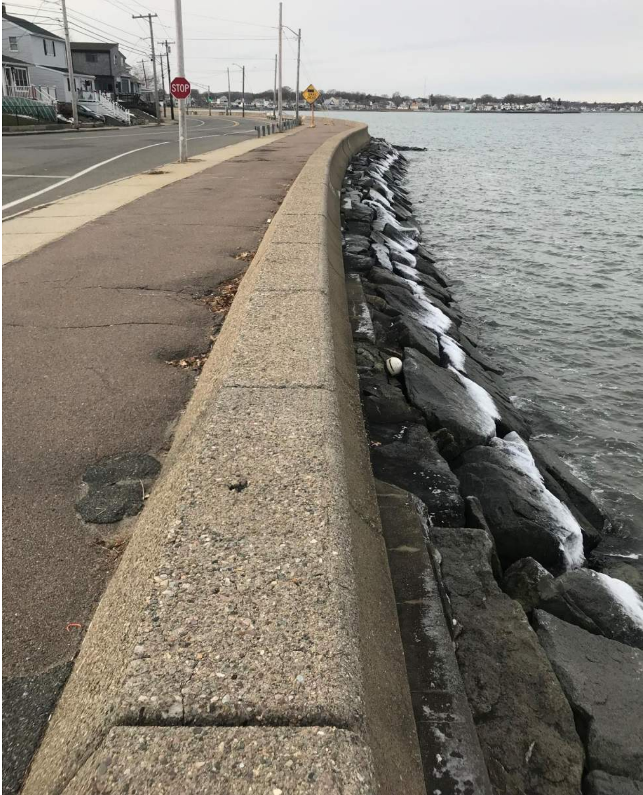
Photo 1: View of the seawall looking west-southwest along Babcock Street toward Sea Street (12/14/17).
