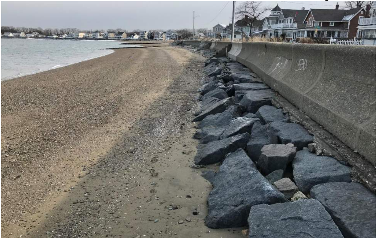
Photo 12: View of seawall and revetment looking east-southeast toward the intersection of Elcott Street and Post Island Road (in top right of photo) (12/14/17).
