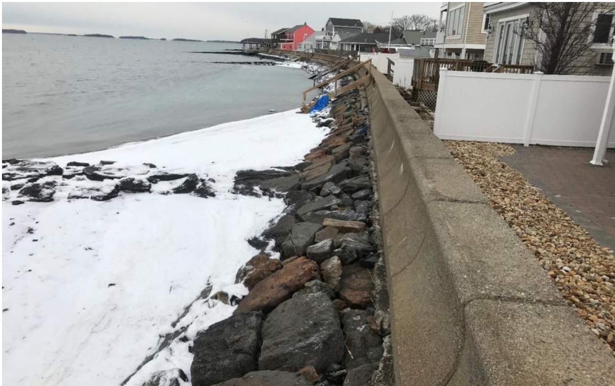
Photo 5: View looking northeast along precast concrete seawall and revetment toward stairs, groins, and the gazebo near OF-02708 (12/14/17).
