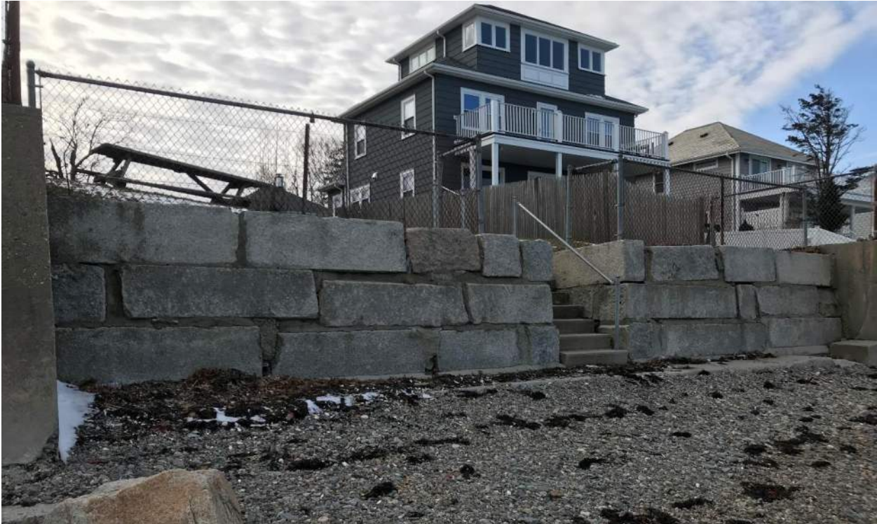
Photo 31: View looking southwest at private concrete block and mortar wall near 54 Norton Road (12/14/17).
