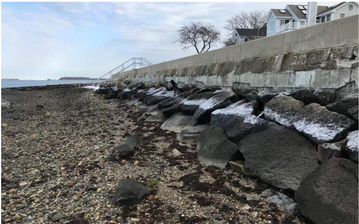
Photo 23: View looking northeast at the precast concrete seawall and revetment, near the intersection of Crane Road and Shellton/Terne Roads (12/14/17).
