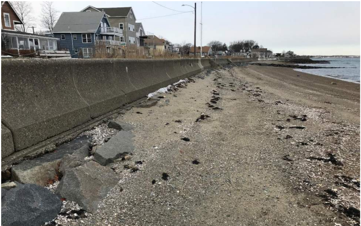
Photo 11: View of the seawall and revetment looking west. Elcott Road intersects Post Island Road in the top left corner of the photo (12/14/17).
