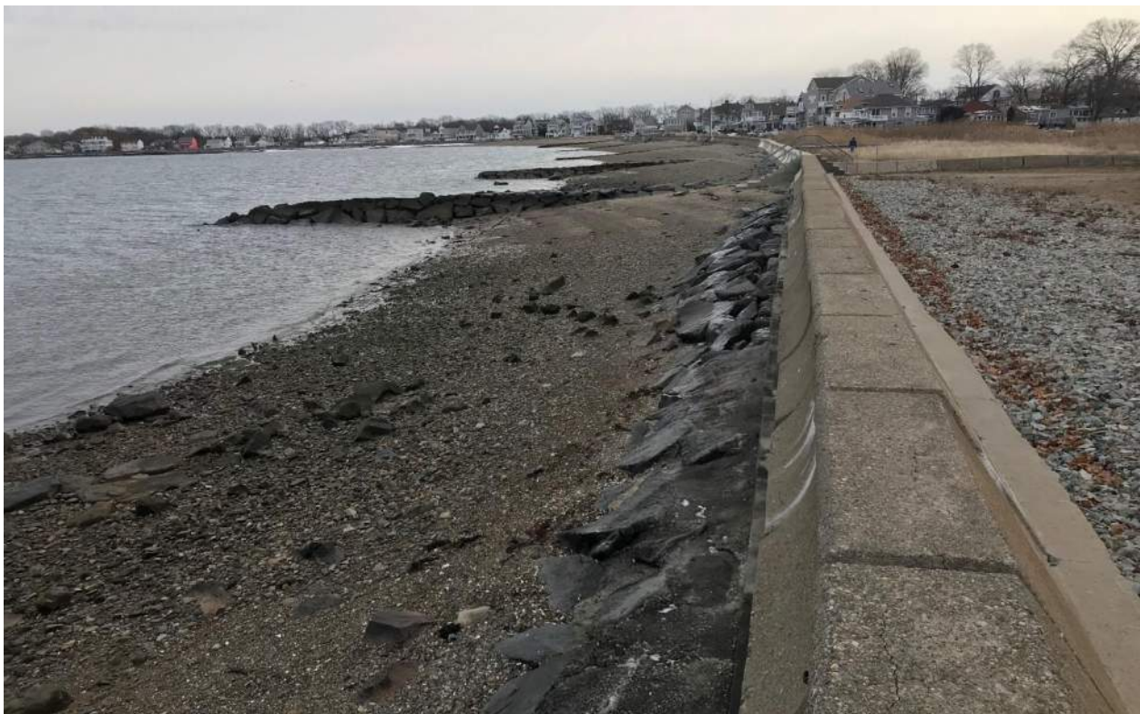
Photo 15: Photo of seawall, revetment, and gravel behind the wall in the area of Arthur Boyson Park, looking east-southeast (12/14/17).
