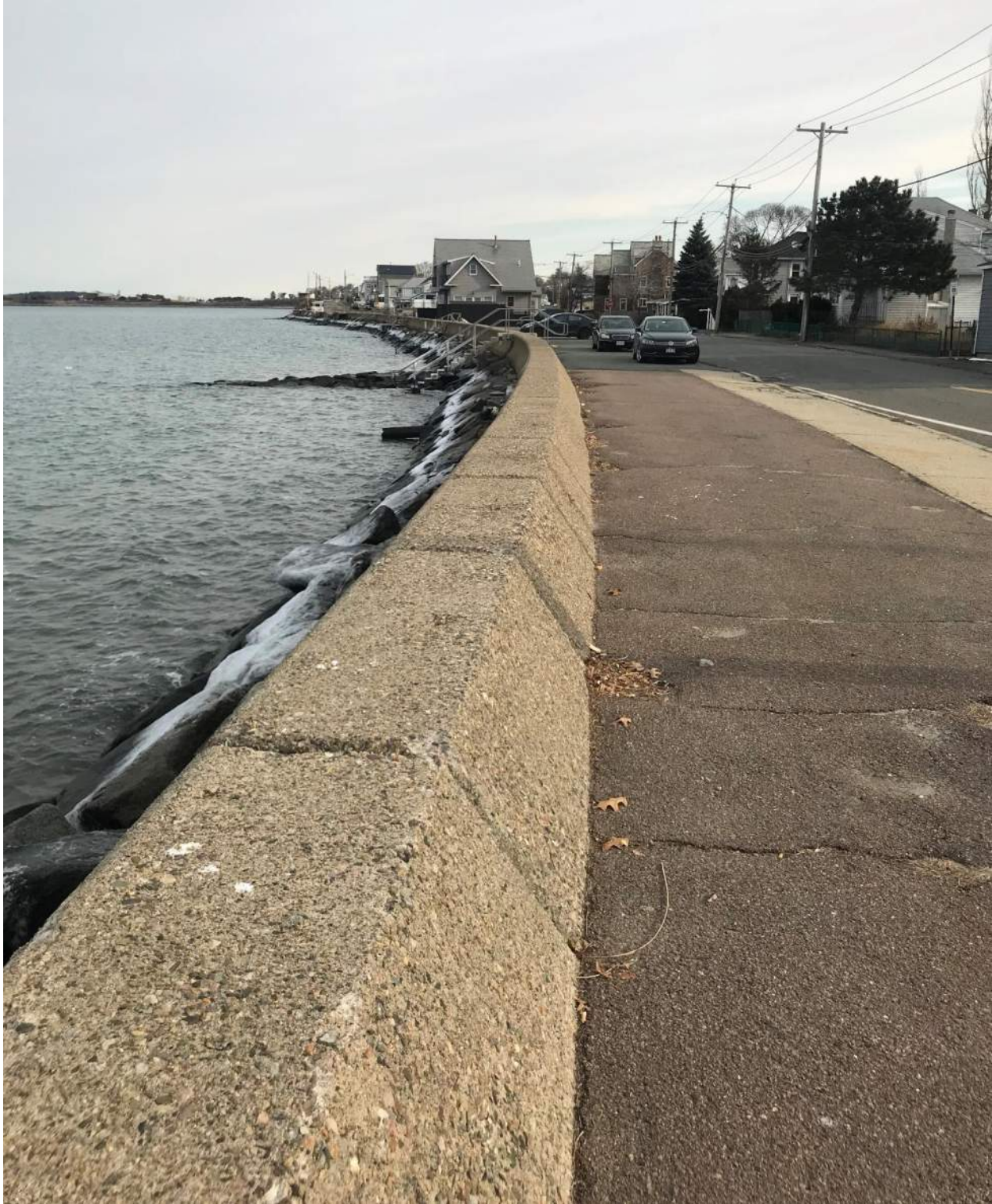
Photo 3: View of precast concrete seawall along Sea Street looking west toward the intersection of Babcock Street and Sea Street (12/14/17).
