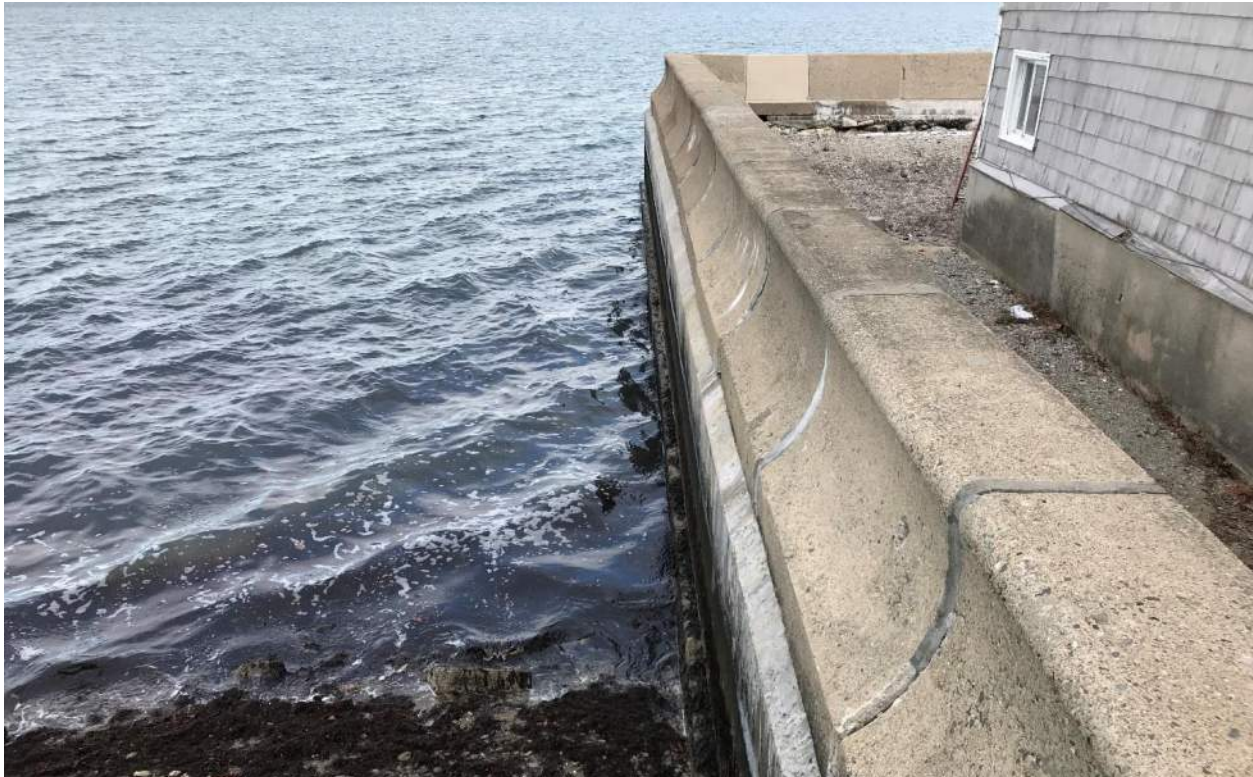
Photo 17: Photo of precast concrete seawall units on top of sheet pile/cast in place wall around 72 Shellton Road, looking north from the southwest corner (12/14/17).
