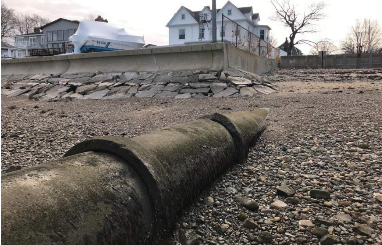
Photo 35: View of outfall OF-08549 (Chickatabot outfall), looking southeast toward the Chickatabot Road, the seawall, and revetment. (12/14/17).
