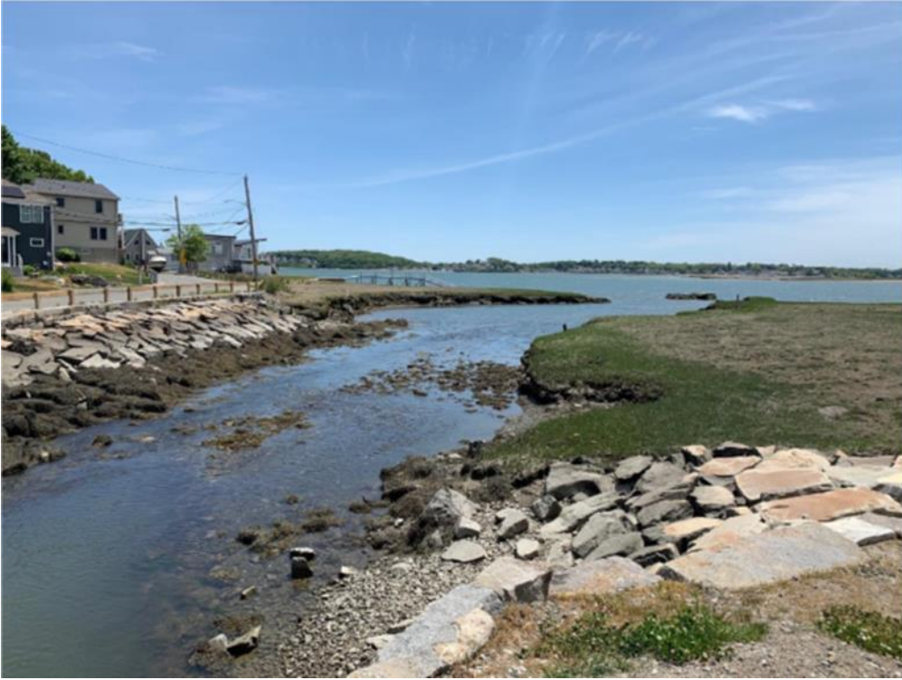
Salt Marsh Down Stream from Rockland Street Culvert
