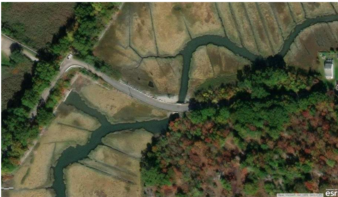
Photo 8: Rhoda Street Crossing Current Conditions
