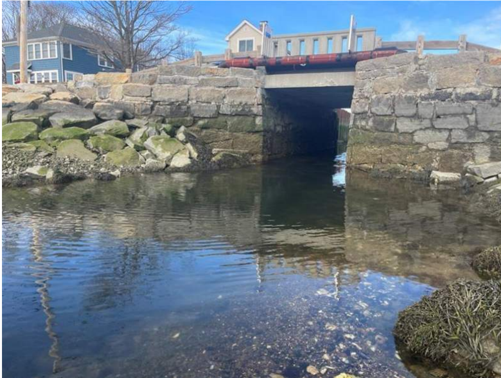
Photo 19: Rockland Street Culvert
