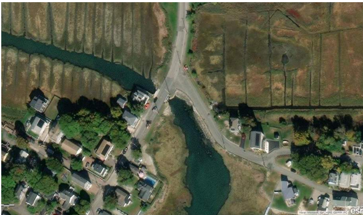
Photo 8: Rhoda Street Crossing Current Conditions
