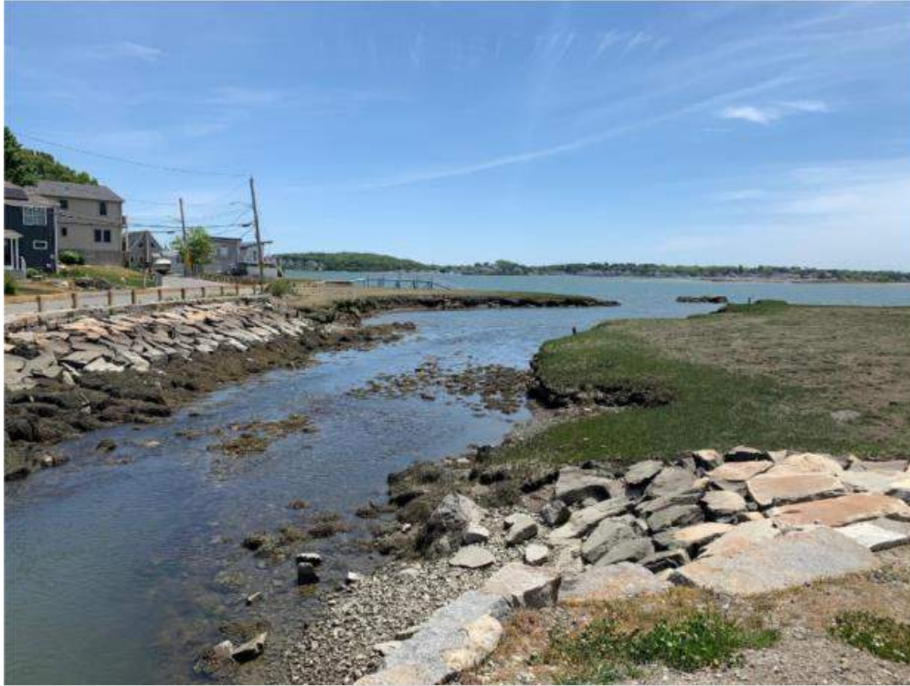
Photo 1: Salt Marsh Down Stream from Rockland Street Culvert
