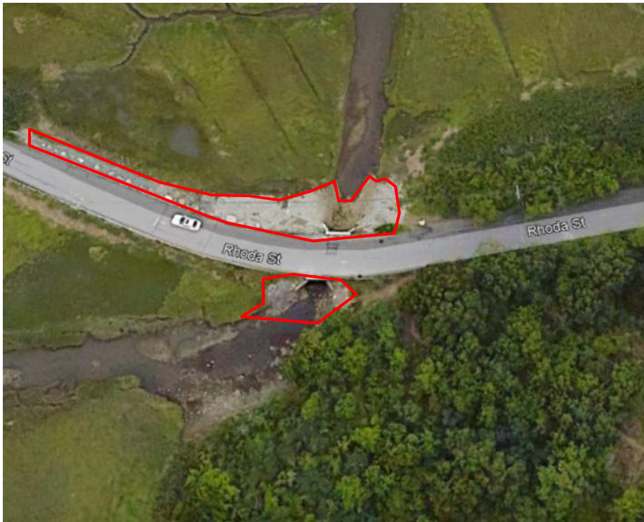
Figure 24: Rhoda Street Culvert Existing Conditions
