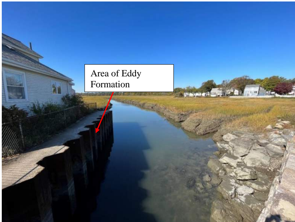
Photo 4: Upstream of Rockland Street Culvert
