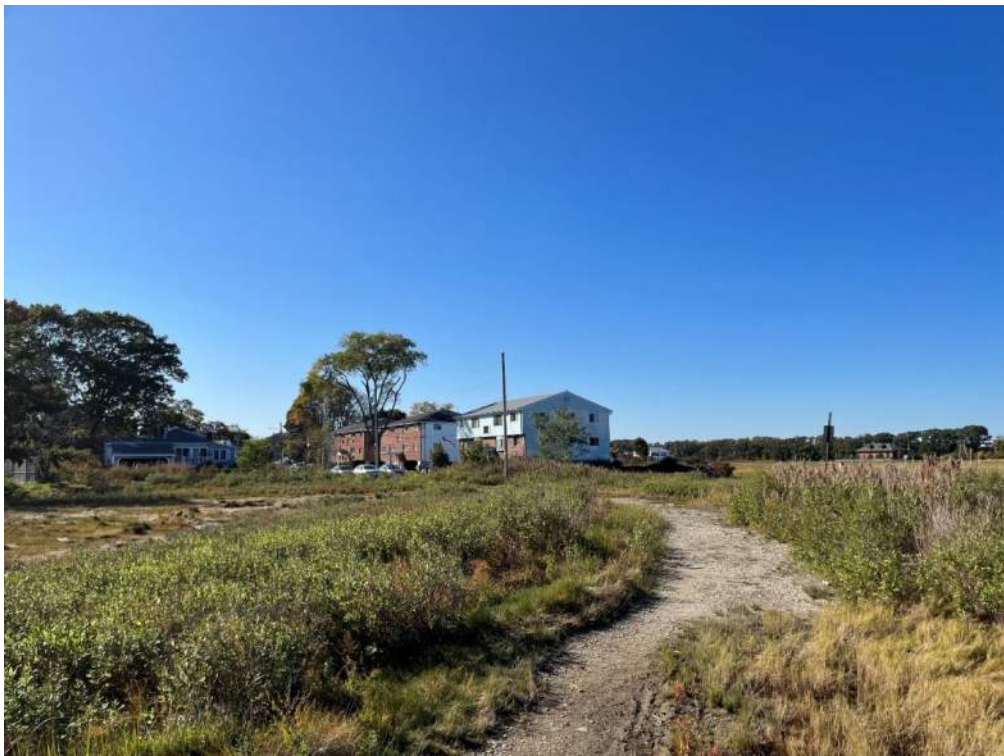
Photo 3: Man Made At-Grade Access Path Adjacent to Lind Street
