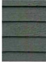
FIBER CEMENT LAP SIDING Material: Fiber Cement Lap Siding 6" Exposure Manufacturer: TBD Color: SW7047 Porpoise
