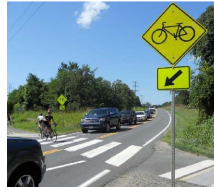
Quality roadway crossings for trails
