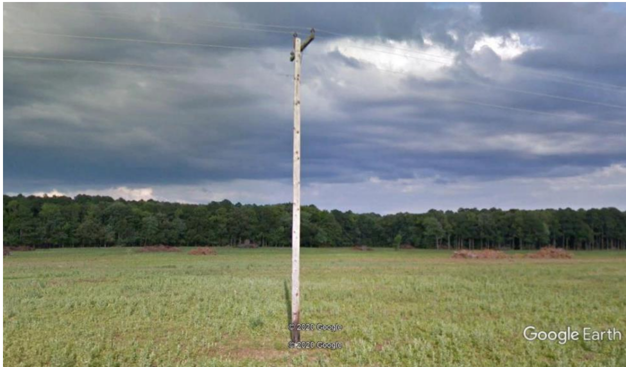
Figure 17: Low-Make-Ready Pole Line in Unserved Area
