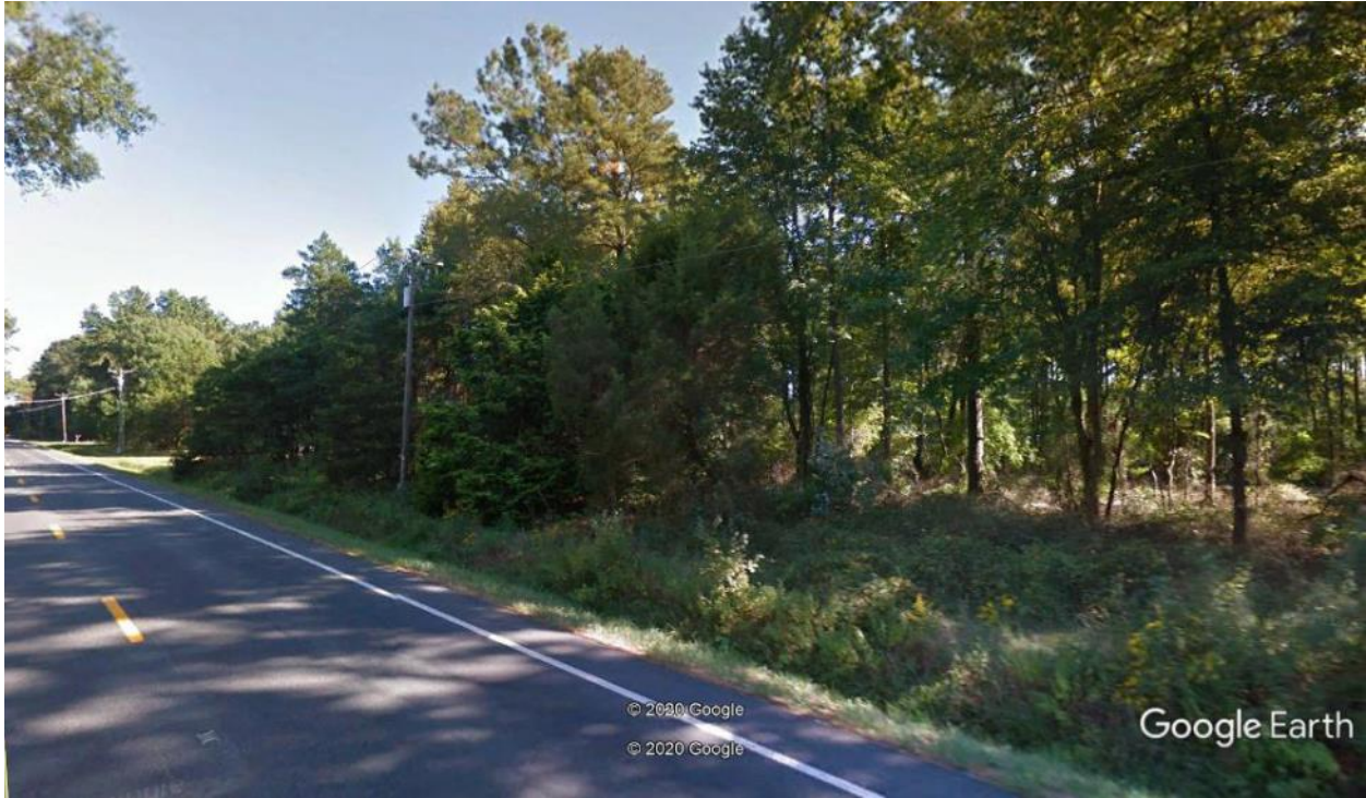
Figure 16: Pole Line Where Tree Trimming Will Be Required
