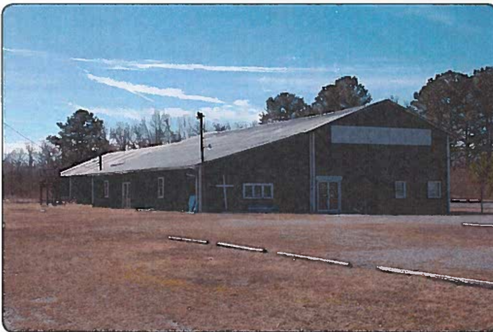
Substation Parcel Perry Road
