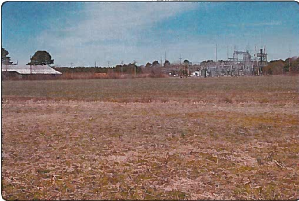
Substation Parcel Perry Road
