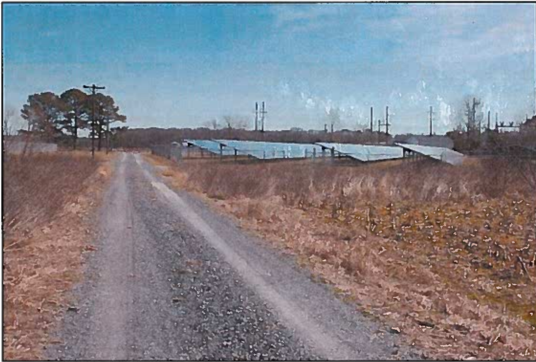
Inset 1. Foreground view of existing PV panels. (Photograph by EDR, March 2015).
