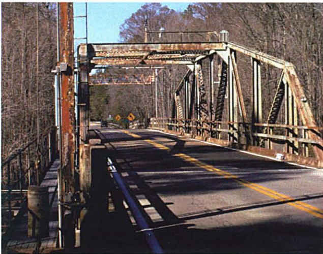
Existing South Quay Bridge over Blackwater River.
