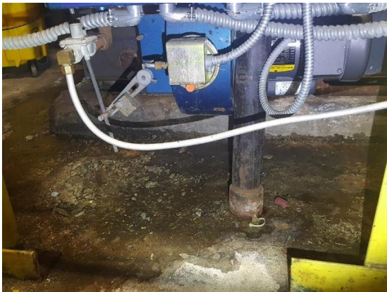
Concrete disintegrating
