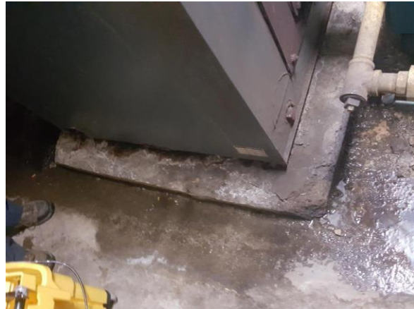
Concrete disintegrating
