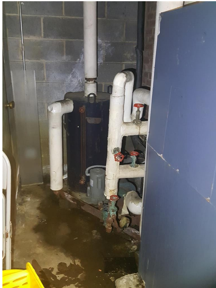
Condensate Receiver and Pump
