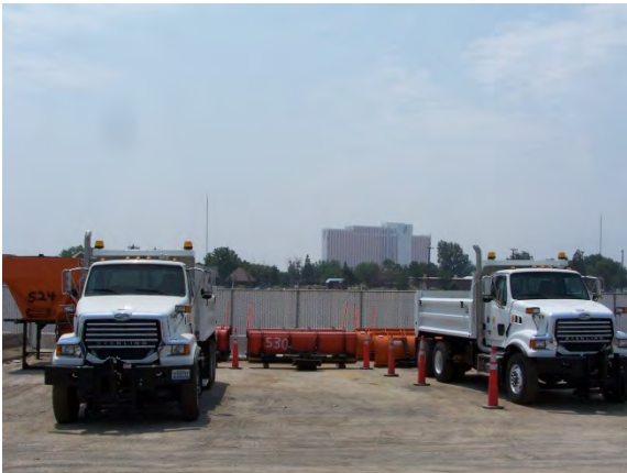
Satellite Site 1 (South 21 st Street)
