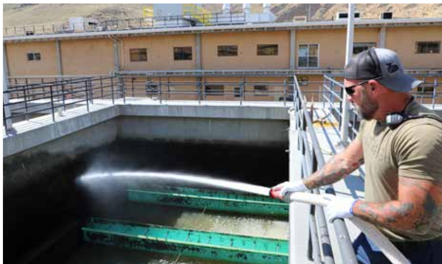
Chris Sneed washes down sand filter cells to keep them clean and filtering well
