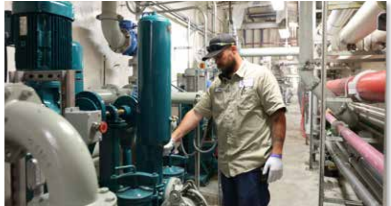
Mechanic Cory Gurr inspects the new diaphragm pump he helped install
